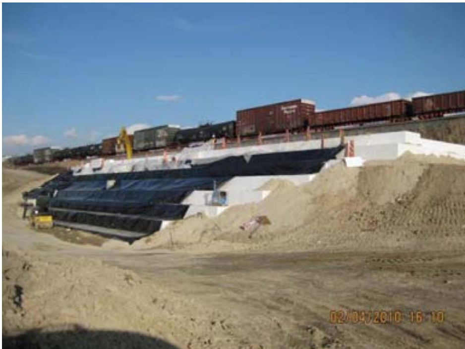
Figure 2.8. Geofoam at UTA FrontRunner Commuter Rail
