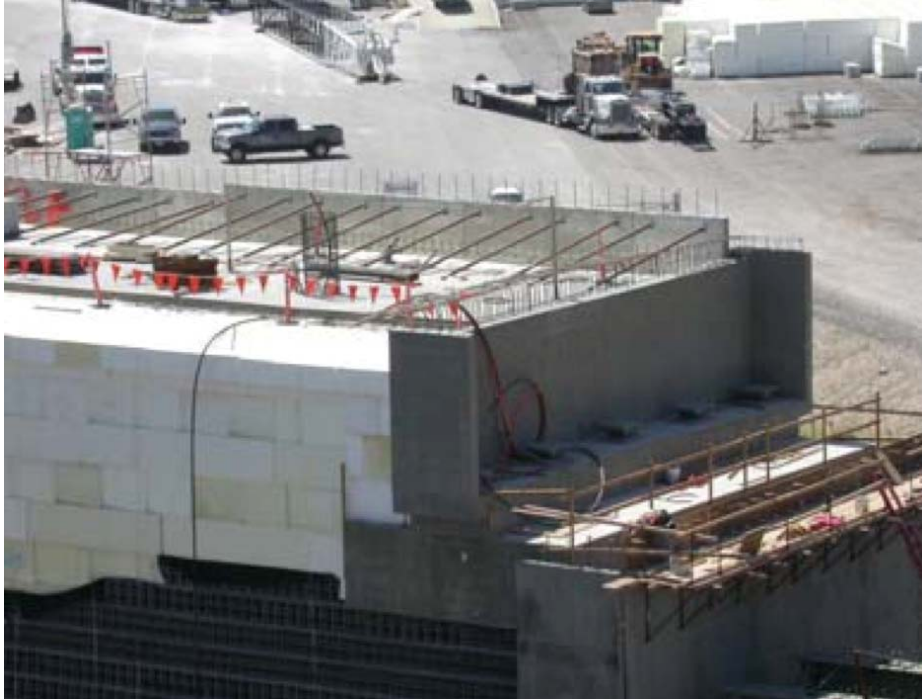
Figure 2.7. Geofoam at UTA TRAX Light Rail
