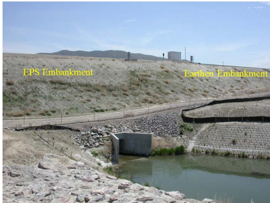
Figure 5.1. Embankment with EPS geofilm and conventional fill materials in Draper city of Utah along FrontRunner line
