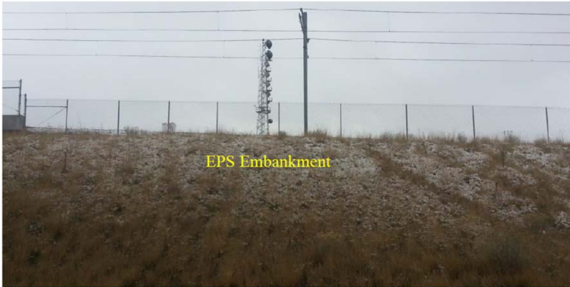
Figure 5.3. EPS embankment to support light rail along Green Line near Roper Yard of Utah
