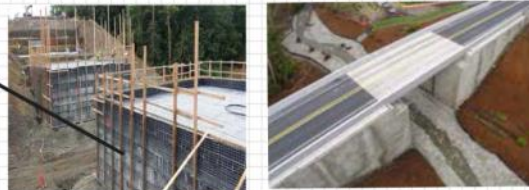
Finished LCC wall with shotcrete
