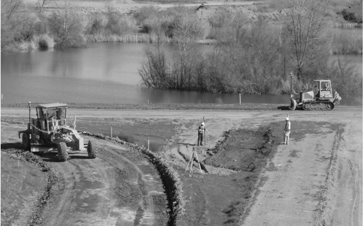
Figure 15.6 A dozer and grader using machine control to create an intersection of roads. (Courtesy Topcon Positioning Systems, Inc.)
