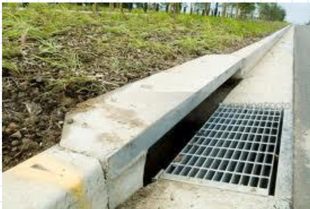
Steel grate over storm drain inlet
