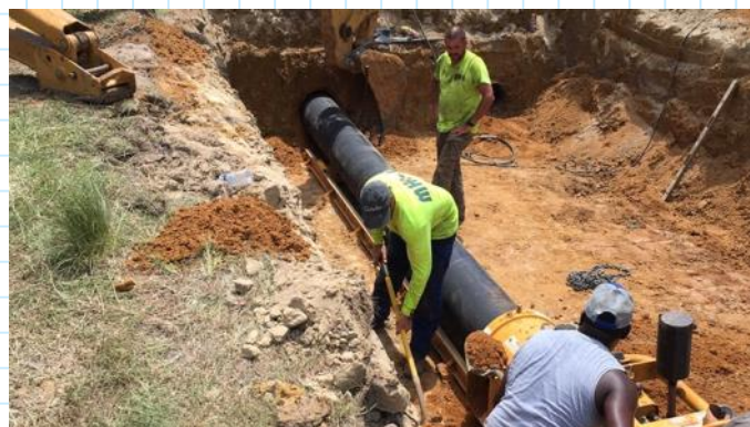
Sewer line installation
