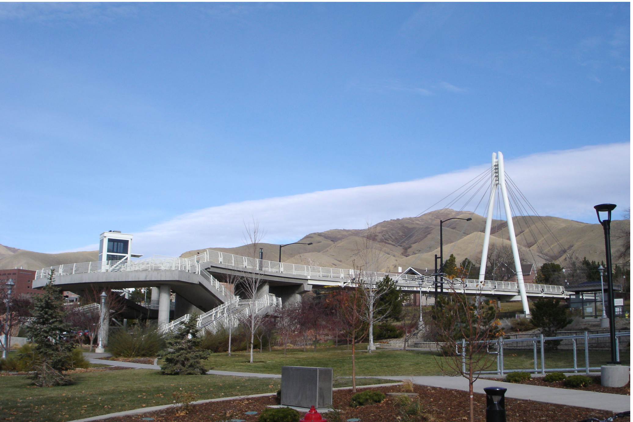
U of U Legacy Bridge
