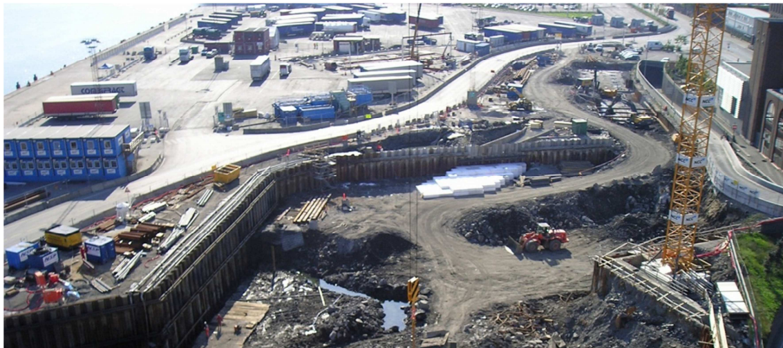
Figure 4: EPS-fill at Havnelageret excavation
