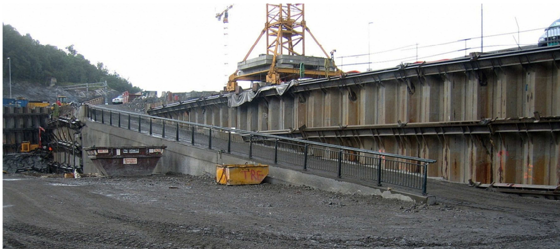
Figure 7: Finished ramp at Sørrenga
