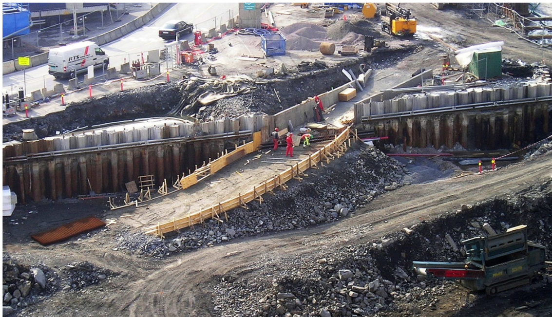
Figure 5: Combination of EPS-fill and concrete ramp at Havnelageret.
