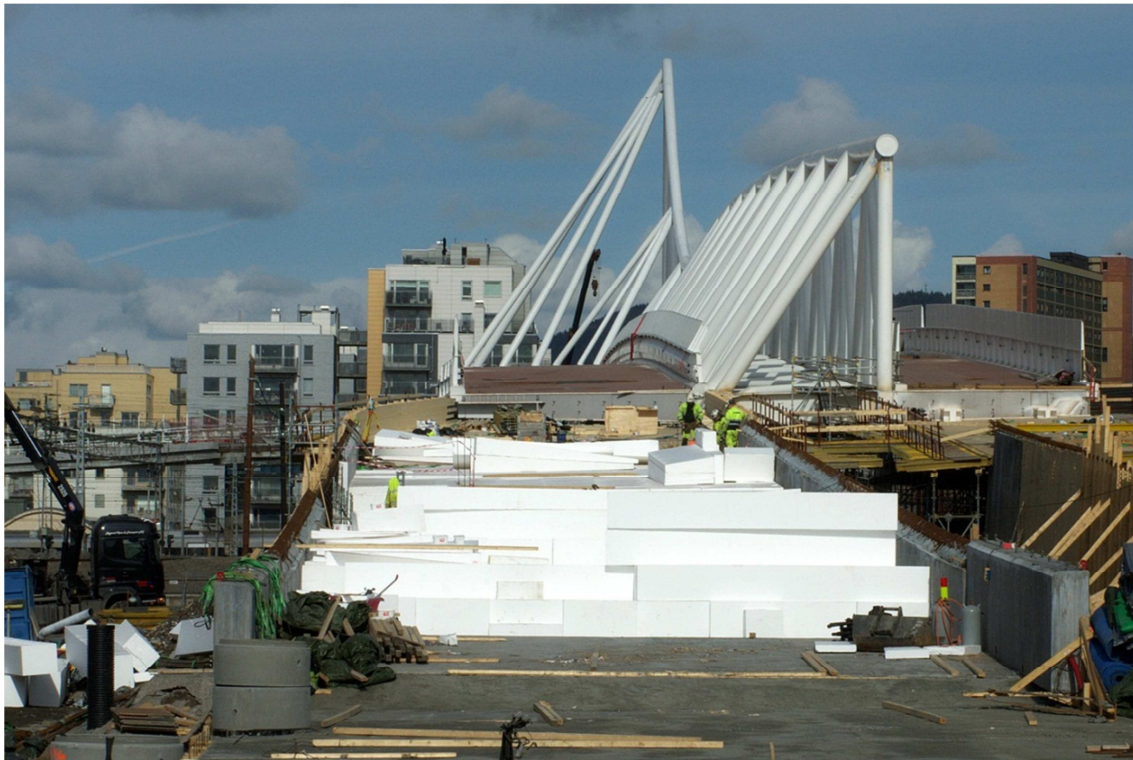
Figure 10: EPS fill for the Nordenga bridge
