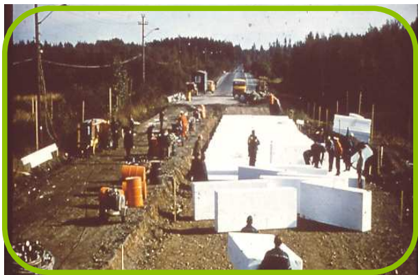
Figure 4. The first layer of EPS geofom blocks are placed.
