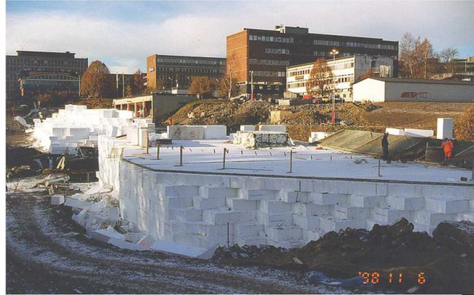
Figure 2. An EPS embankment for a city tramline in Oslo with vertical walls as an alternative to a bridge.
