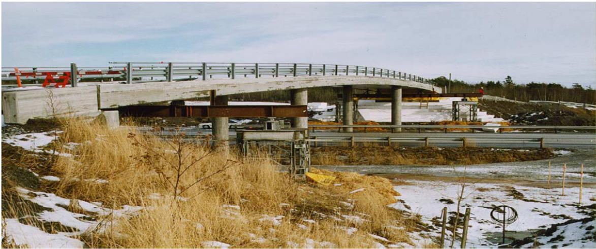
*Figure 19. Temporary support of abutments at Hjelmungen*
