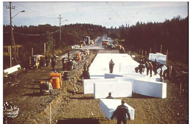
Figure 1. EPS used as lightweight fill material.
