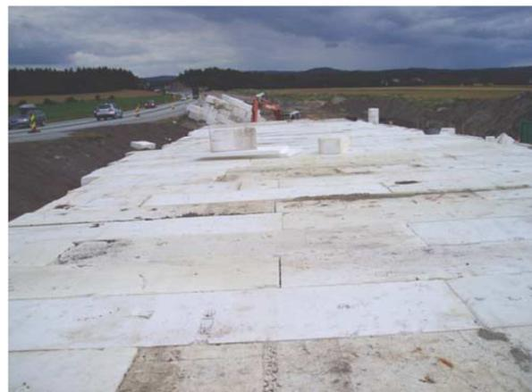
Figure 7 Reuse of EPS blocks from Løkkeberg Bridge
