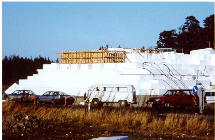
Figure 11. Construction of one abutment on the EPS embankments at Løkkeberg Bridge.
