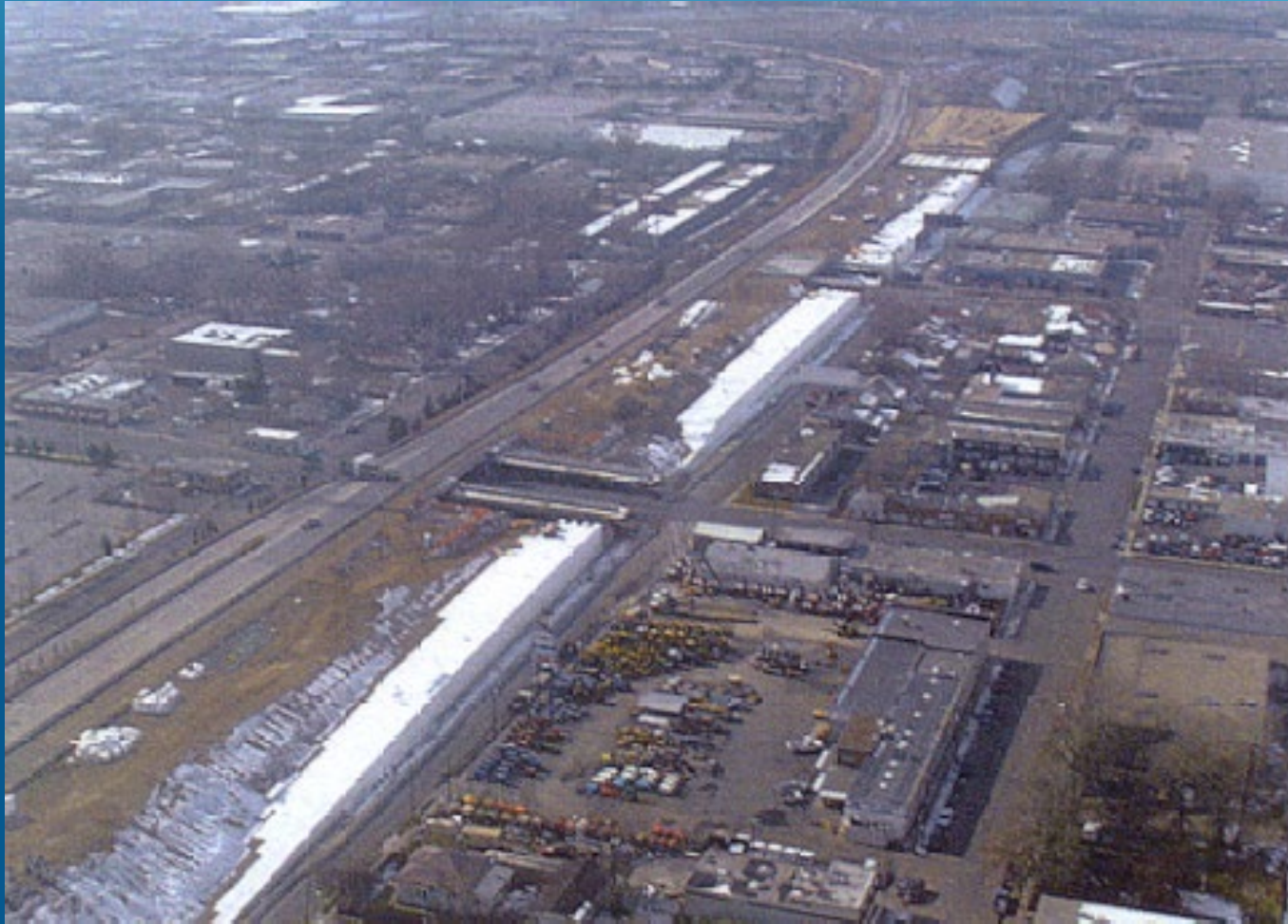
I-15 Reconstruction Project, Salt Lake City, Utah
