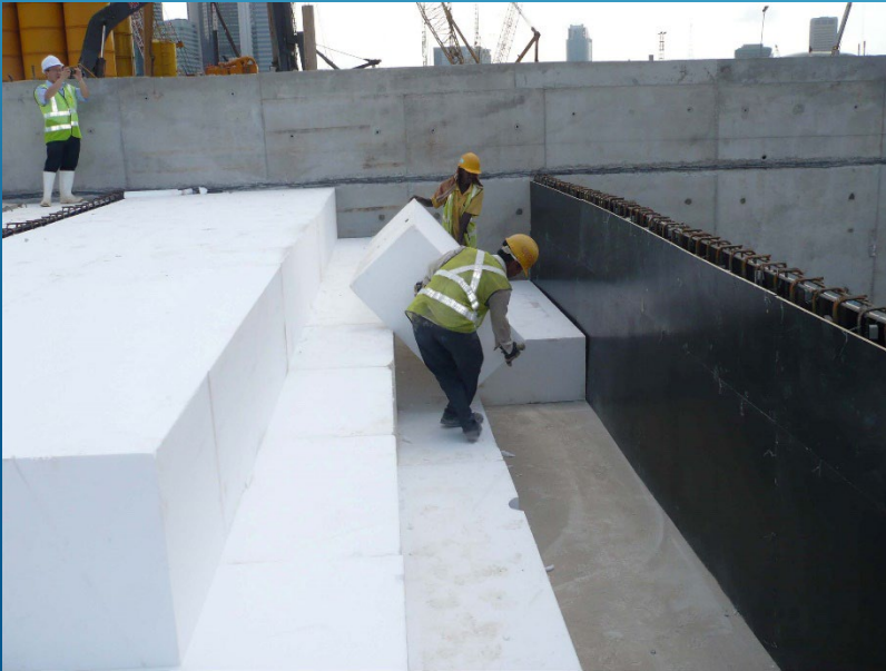
Geofoam Placement photo courtesy of BASF- Kuala Lumpur, Malaysia
