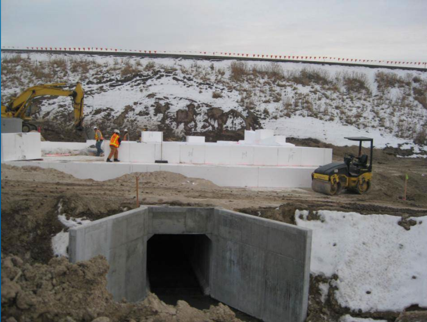
UTA Commuter Rail Widening Over Existing Culvert, Corner Canyon, Draper, Utah
