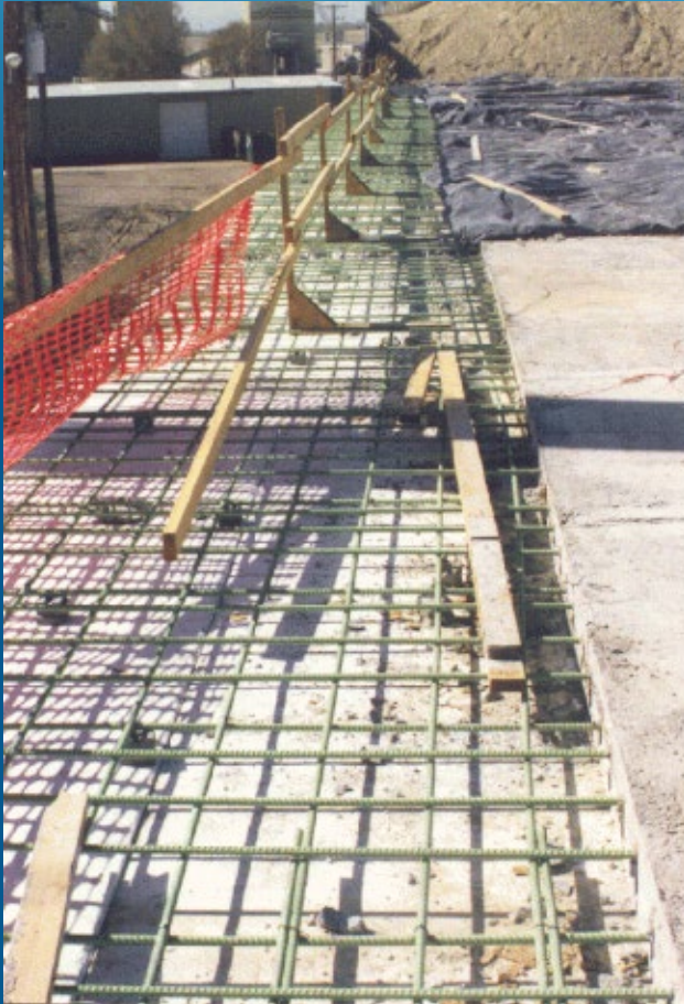
Reinforced Concrete Load Distribution Slab
