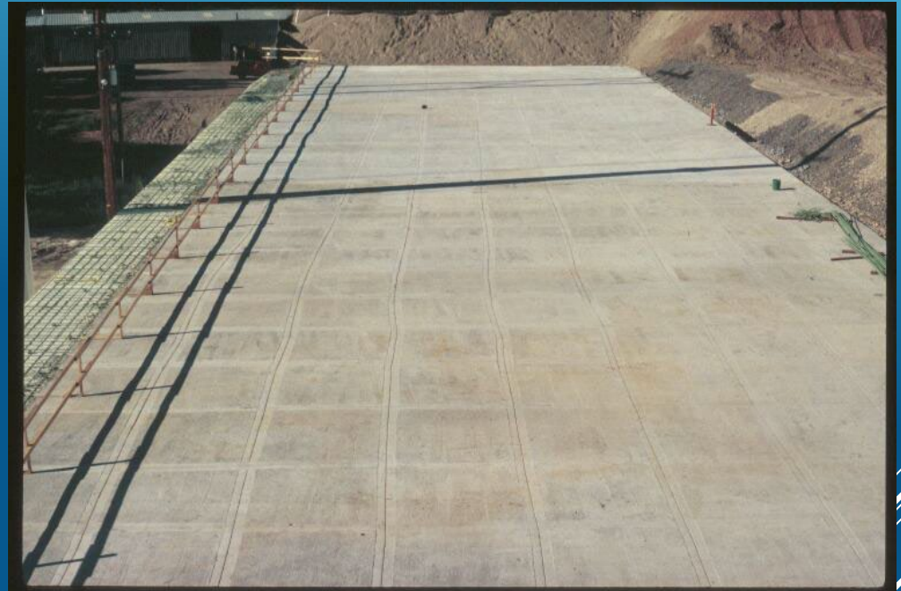
Completed Load Distribution Slab
