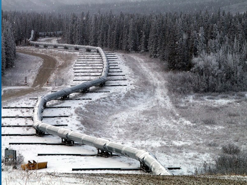
Alaskan Pipeline – Strike Slip Fault
