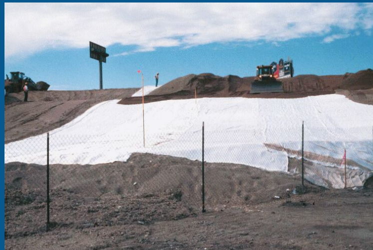
Geotextile Reinforced Slopes
