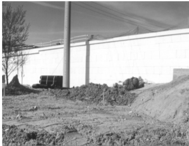
Figure 2: A Geofoam Embankment at 100 South Utility Corridor Crossing of I-15.
