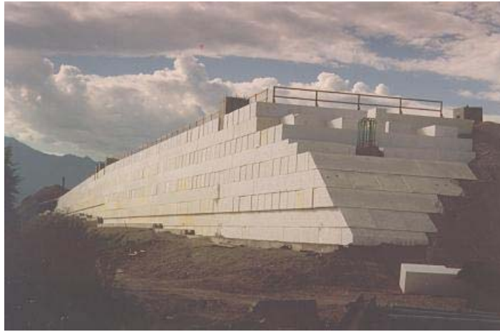
Vertical EPS geofoam embankment fill.
