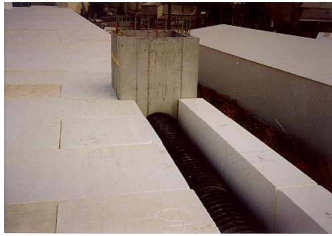
EPS geofoam fill adjacent to storm drain.
