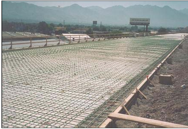
Load Distribution Slab Reinforcement.
