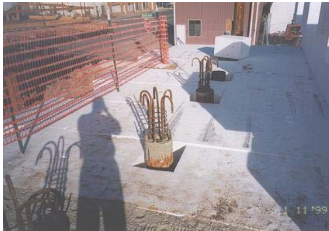
Bridge pier extending through EPS geofoam fill.
