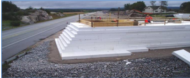
Figure 6. Gimsøyveien bridge during construction
