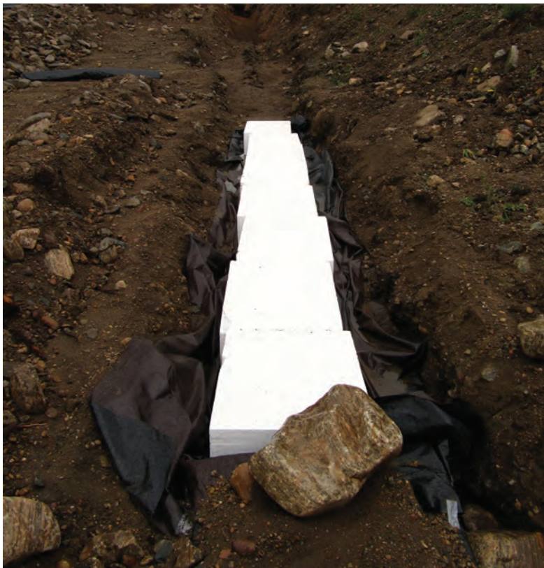
The reduction in loading and deformation due to geofoam's compressibility likely will improve the performance of this Weber Canyon pipeline during and after a major seismic event along the fault area.
