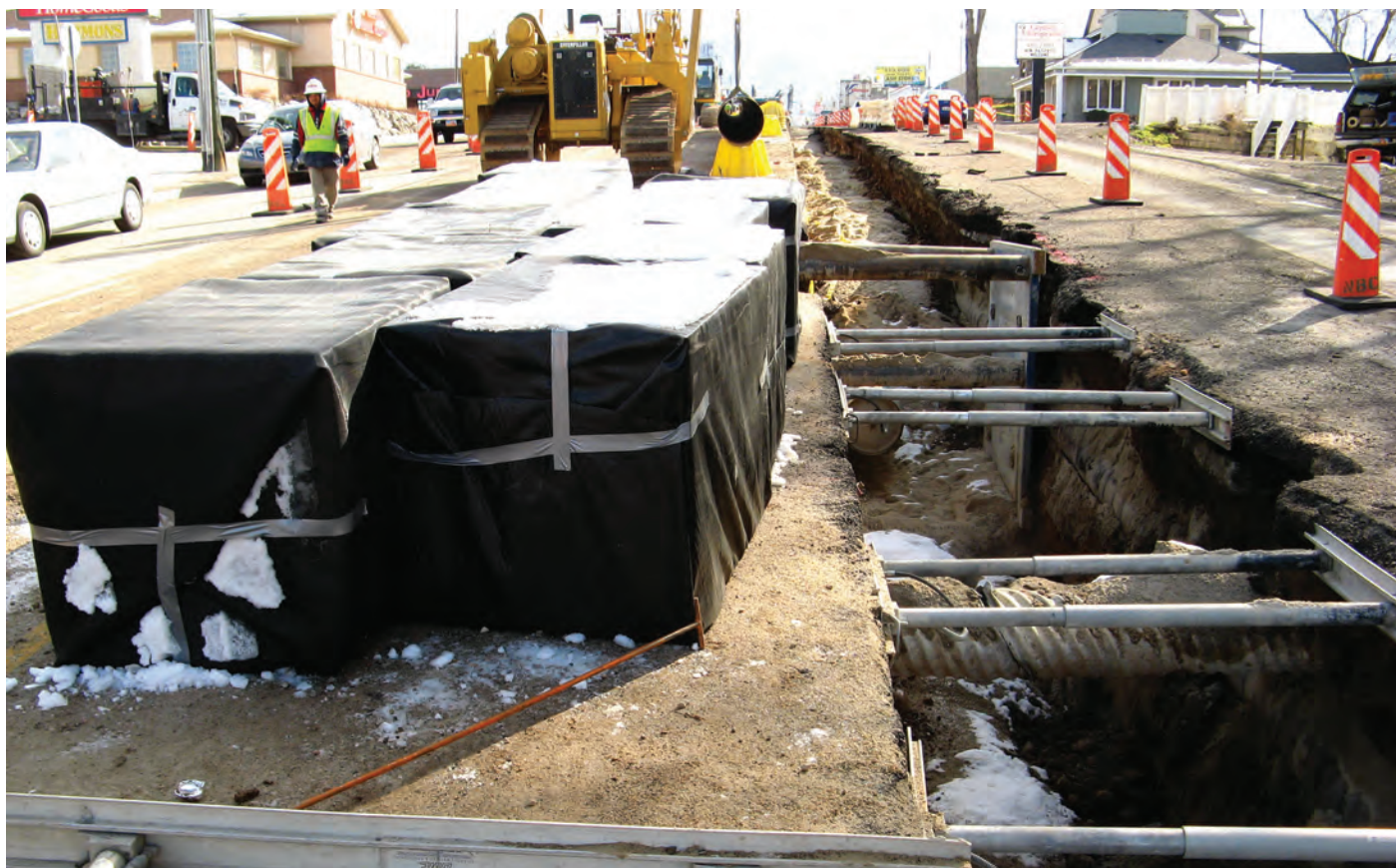
Figure 3: Lightweight geofoam cover system for pipelines. Drawing: Bret Nills Lingwall, University of Utah
