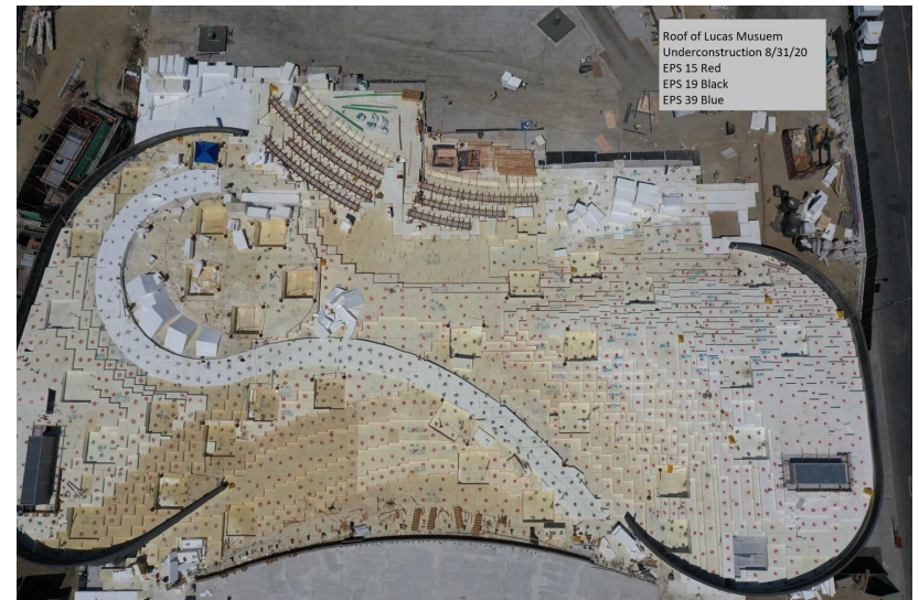
EPS Placement Lucas Museum Los Angeles California – Over Parking Structure
