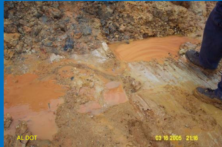
Water at Bottom of Cut
