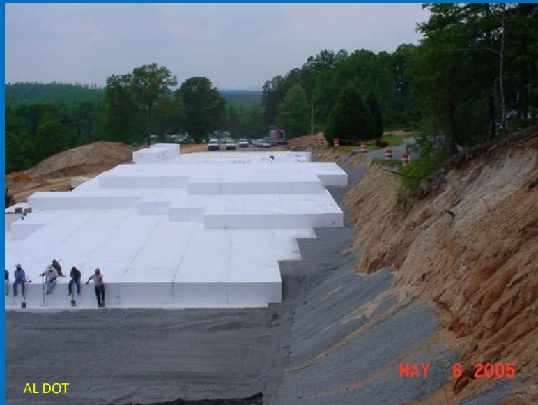
Overview of EPS Block Placement Configuration
