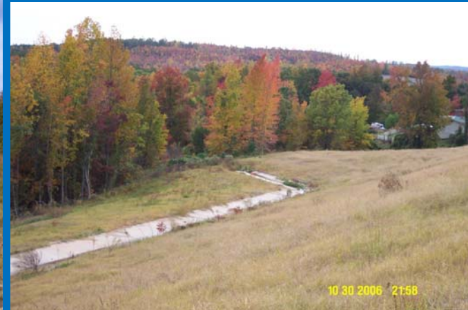
Drainage Channel Diverts Water Away From Slope
