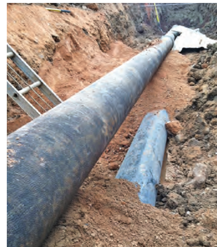
The new ductile iron pipe with locking gaskets is shown above the old abandoned line.
