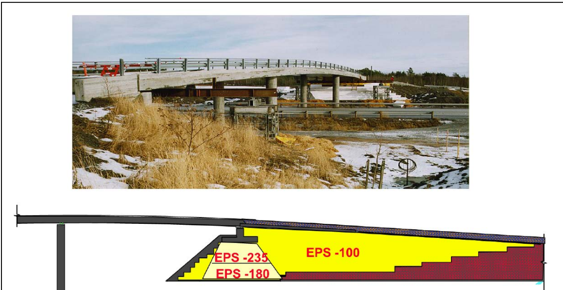
Figure 1-2 Single-lane, single-span, concrete bridge structure supported on EPS block abutment at Hjelmungen, Norway (Aabøe and Frydenlund, 2011).
