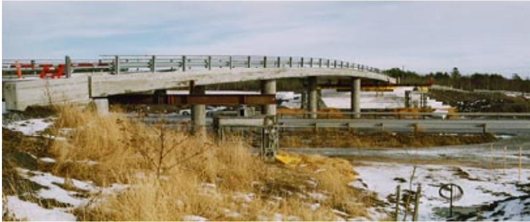
Figure 20: Temporary support of abutments at Hjelmungen.
