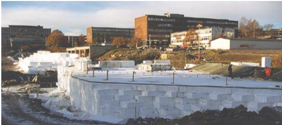
Figure 1: An EPS embankment with vertical walls for a city tramline in Oslo as an alternative to a bridge.
