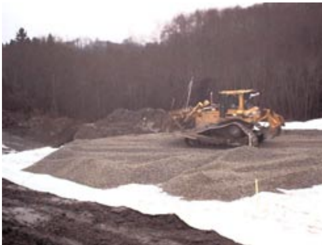
Figure 12: Distribution and compaction with dozer.
