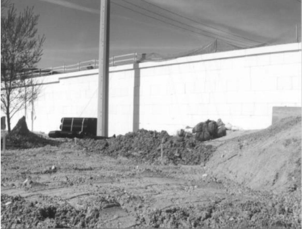
**Figure 2. A Geofoam Embankment at 100 South Utility Corridor Crossing of I-15.**
