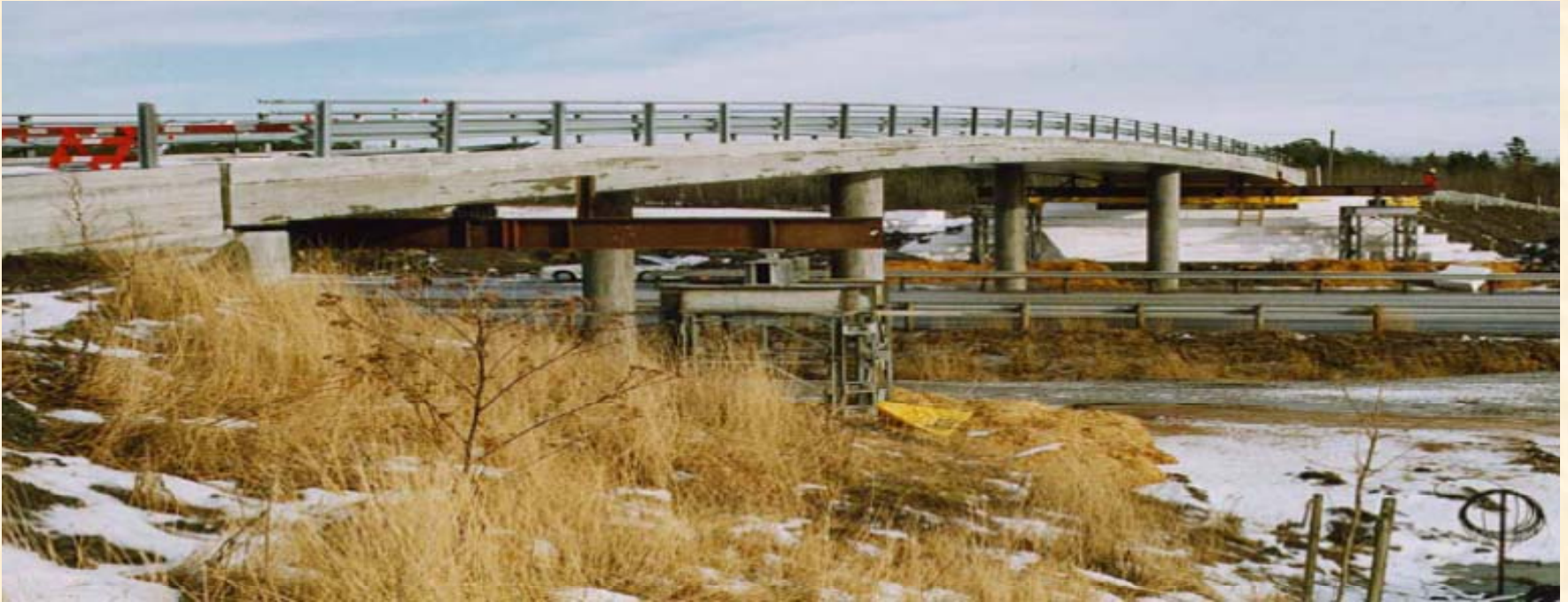
Hjelmungen Bridge, Norway
