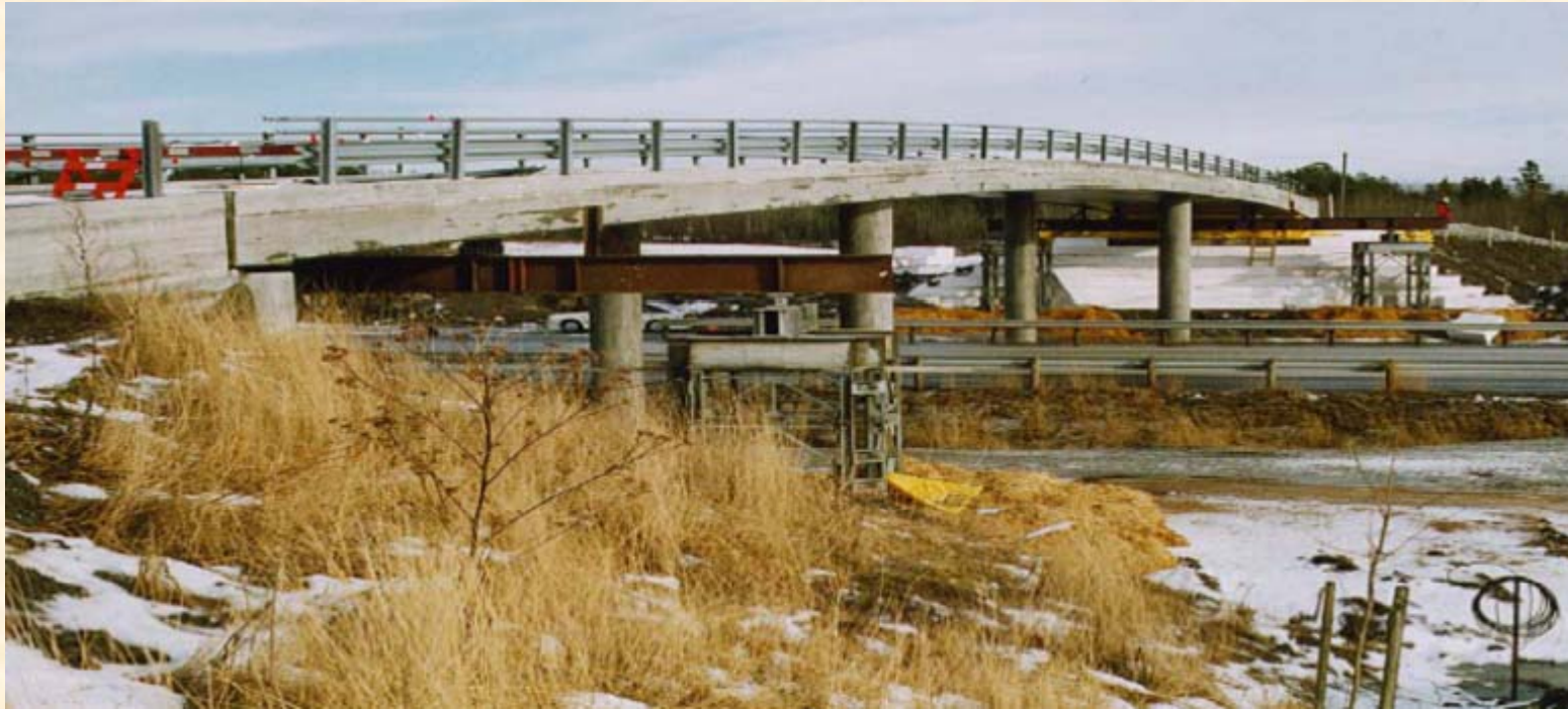
Hjelmungen Bridge, Norway
