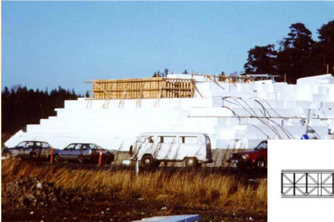
Lokkeberg Bridge, Norway
