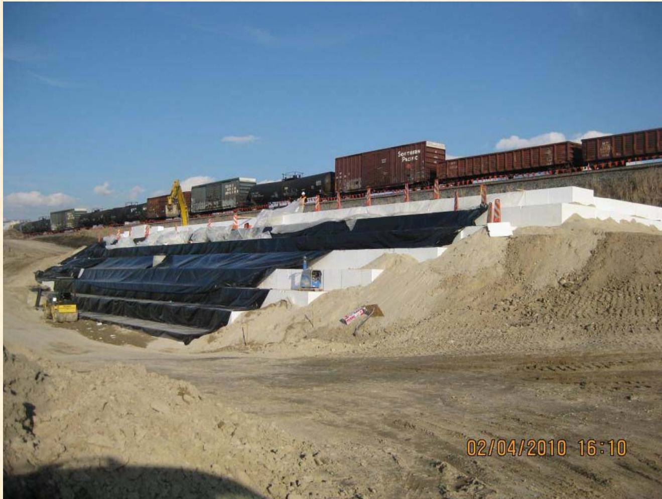
Protection of side slope, UTA Frontrunner, Corner Canyon
