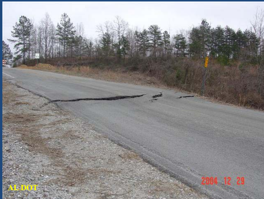
Pavement Cracking
