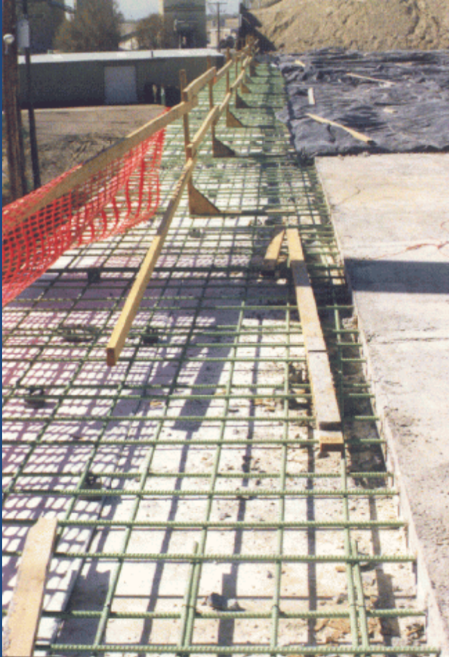
Reinforced Concrete Load Distribution Slab
