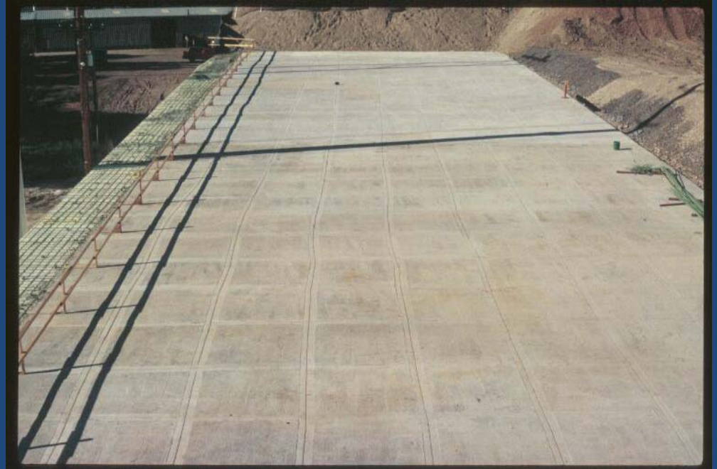
Completed Load Distribution Slab
