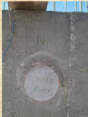
Pressure Cell Cast in Bridge Abutment
