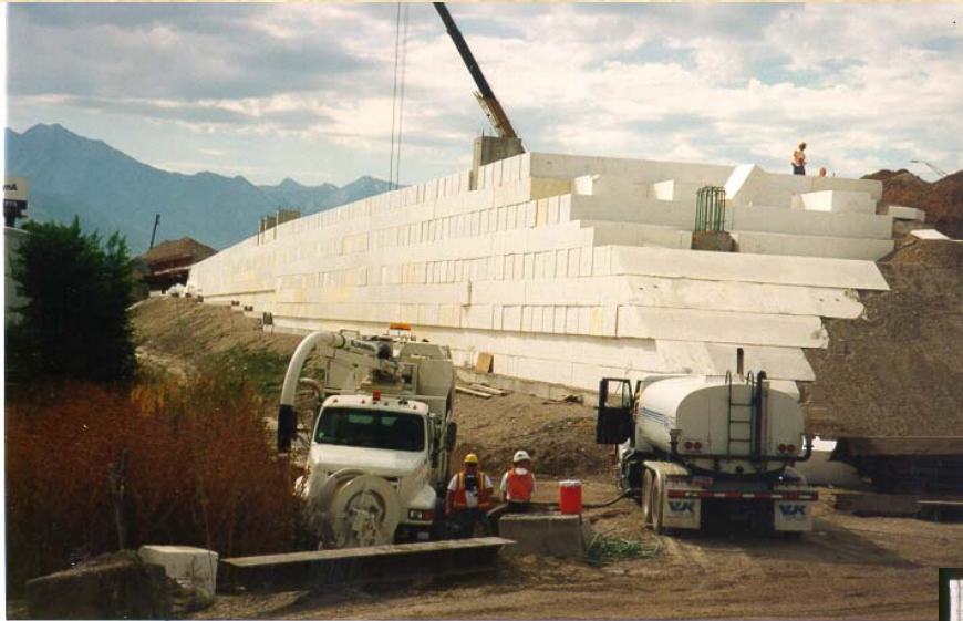
Nearly Completed Geofoam Embankment with Vertical Face
