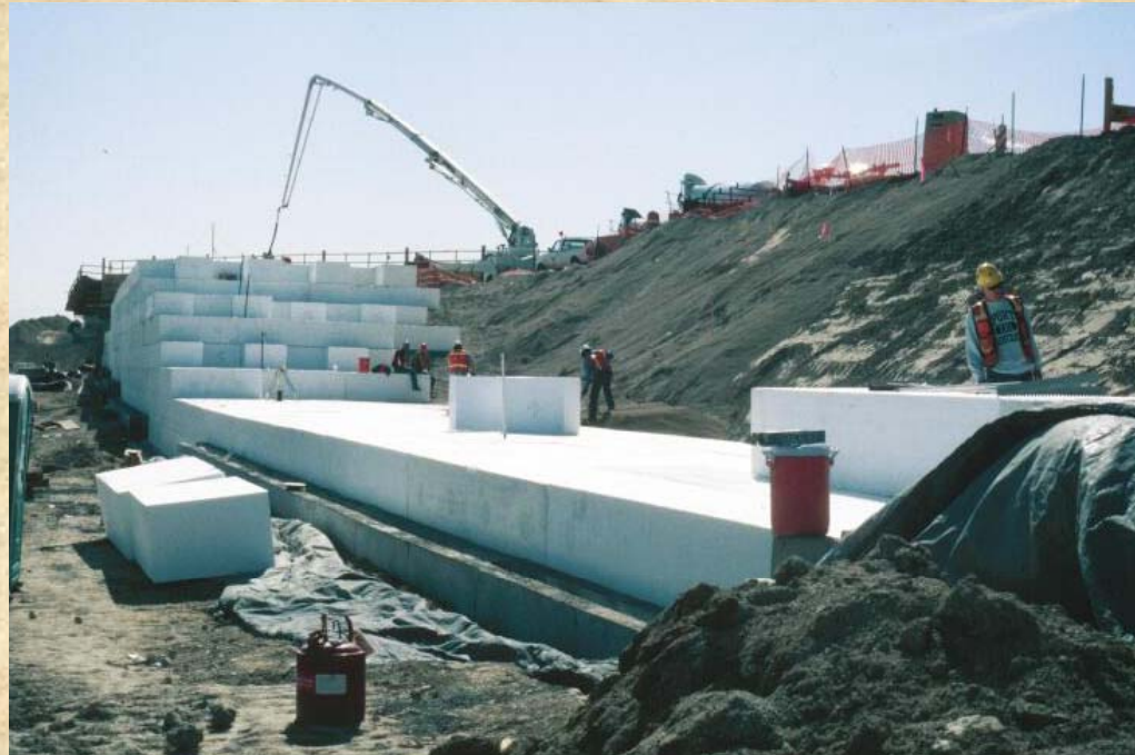
Construction of Geofoam Embankment and Footing for Tilt-up Panel Wall
