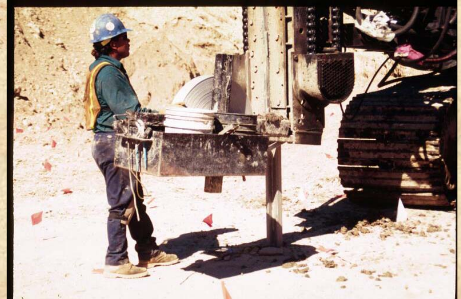
PV drain pushed into ground
