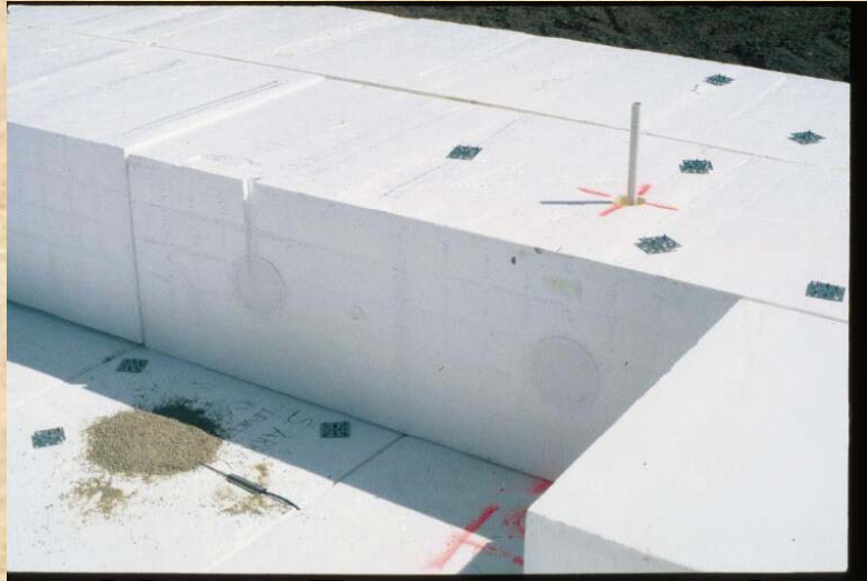
Magnet Extensometer and Pressure Cell Installation
