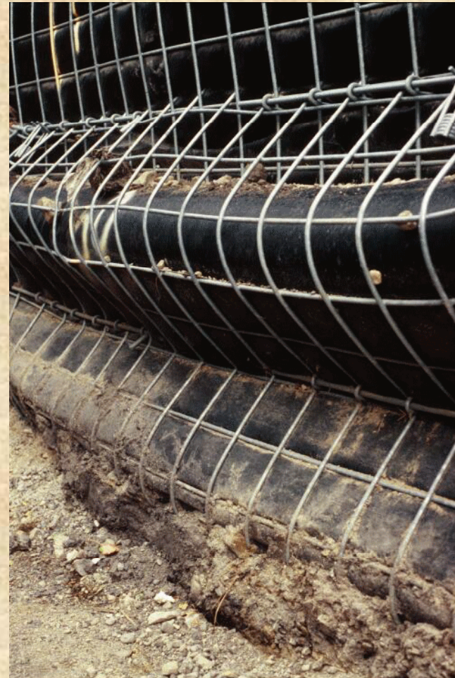
Deformation of Welded Wire Face at Toe of Wall
