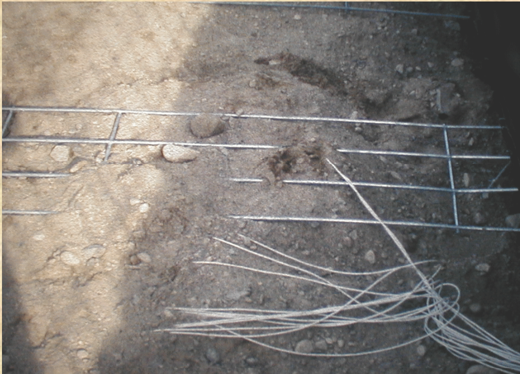
Horizontal reinforcing (bar mat) with strain gages.
