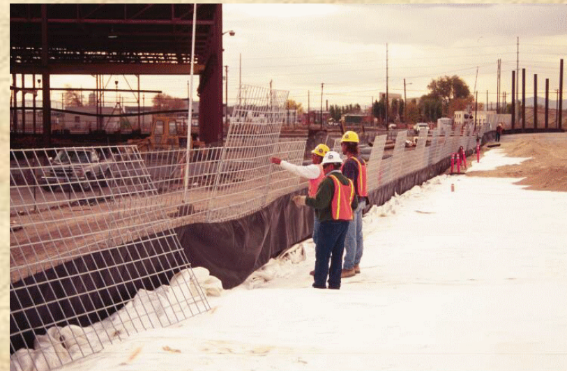
Geotextile lapped into MSE wall
