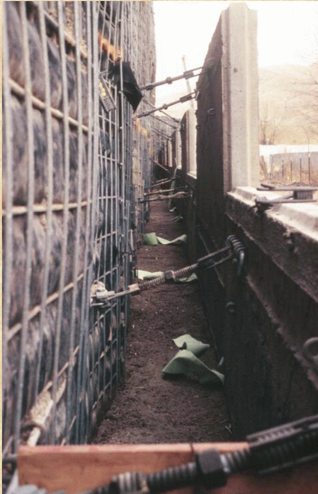
Attachment of Panels with threaded rod
