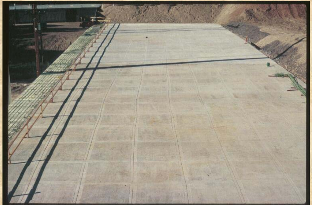
Completed Load Distribution Slab
