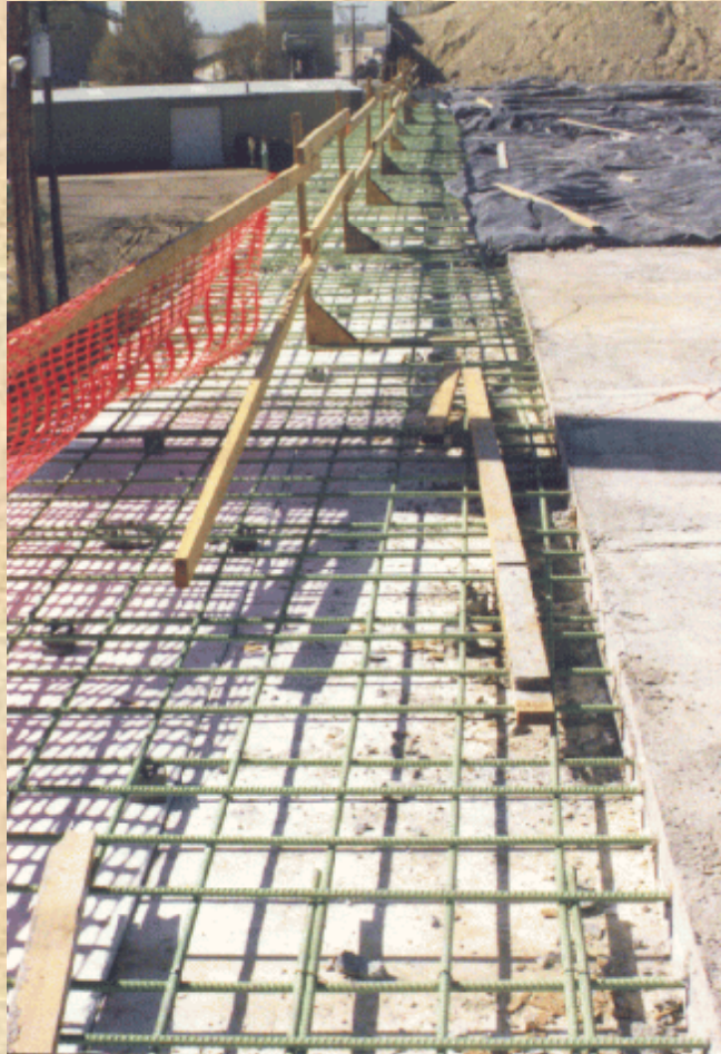
Reinforced Concrete Load Distribution Slab atop Geofoam
