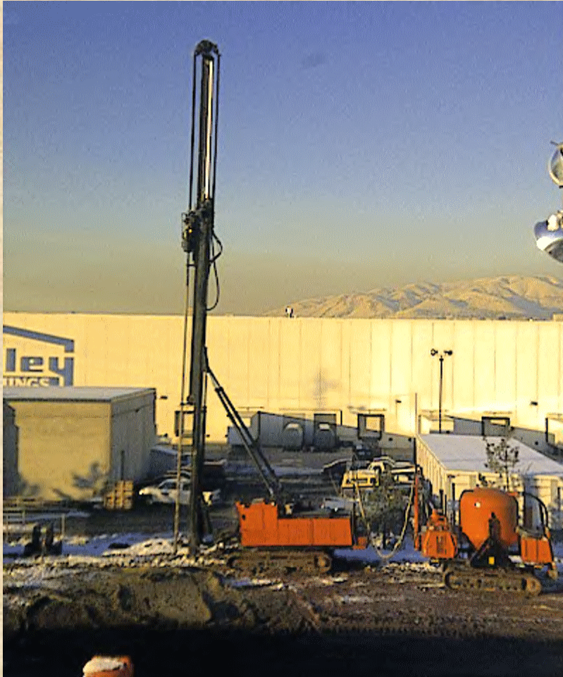
Lime Cement Column Rig
