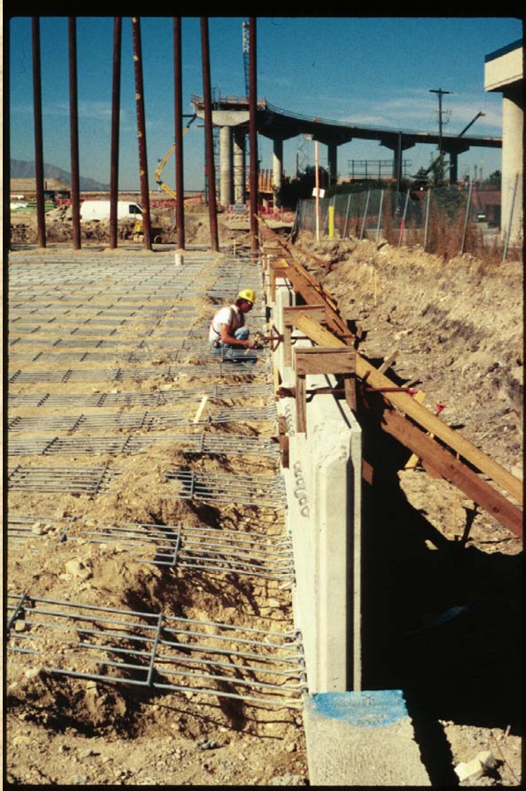
1-stage MSE placed over columns
