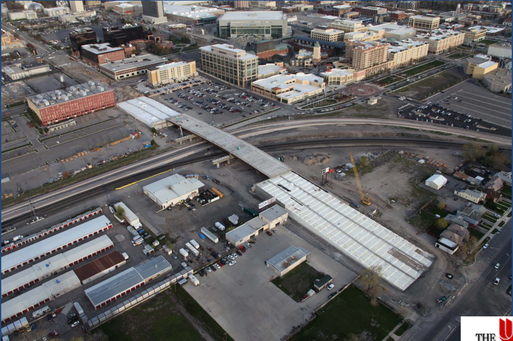
North Temple Viaduct – Salt Lake City, Utah
