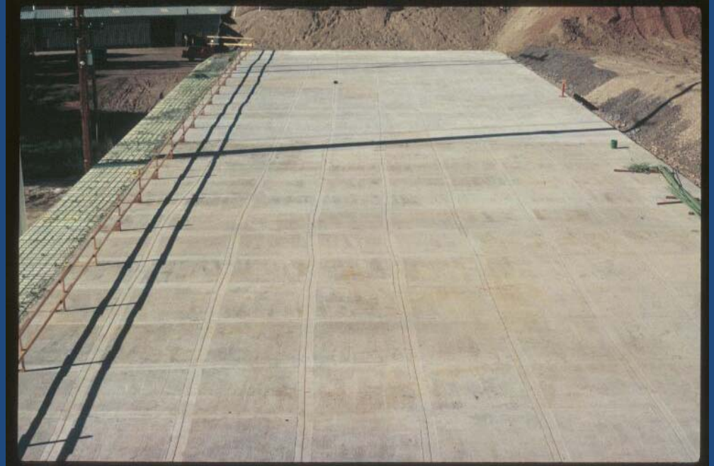
Completed Load Distribution Slab
