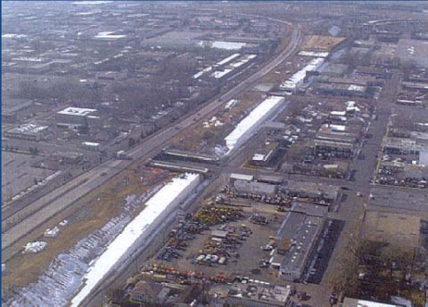
Geofoam Embankment, Salt Lake City, Utah
