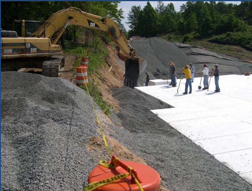
Backfill Placement Behind EPS
