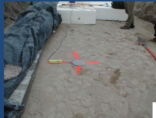
Pressure Cell in Base Sand
