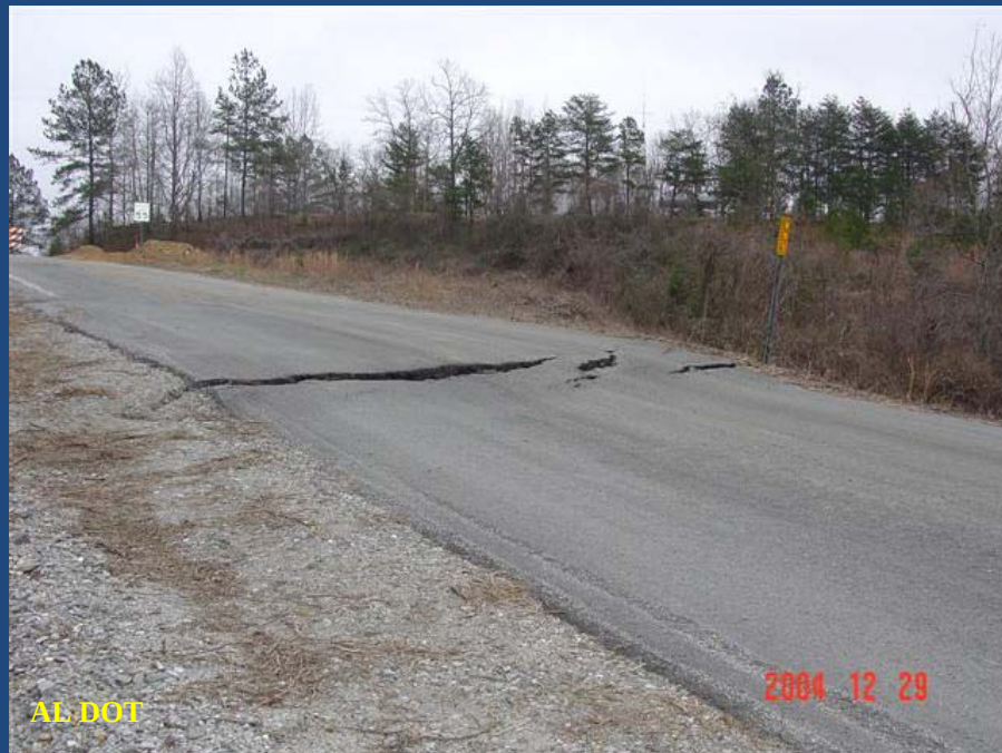
Pavement Cracking
