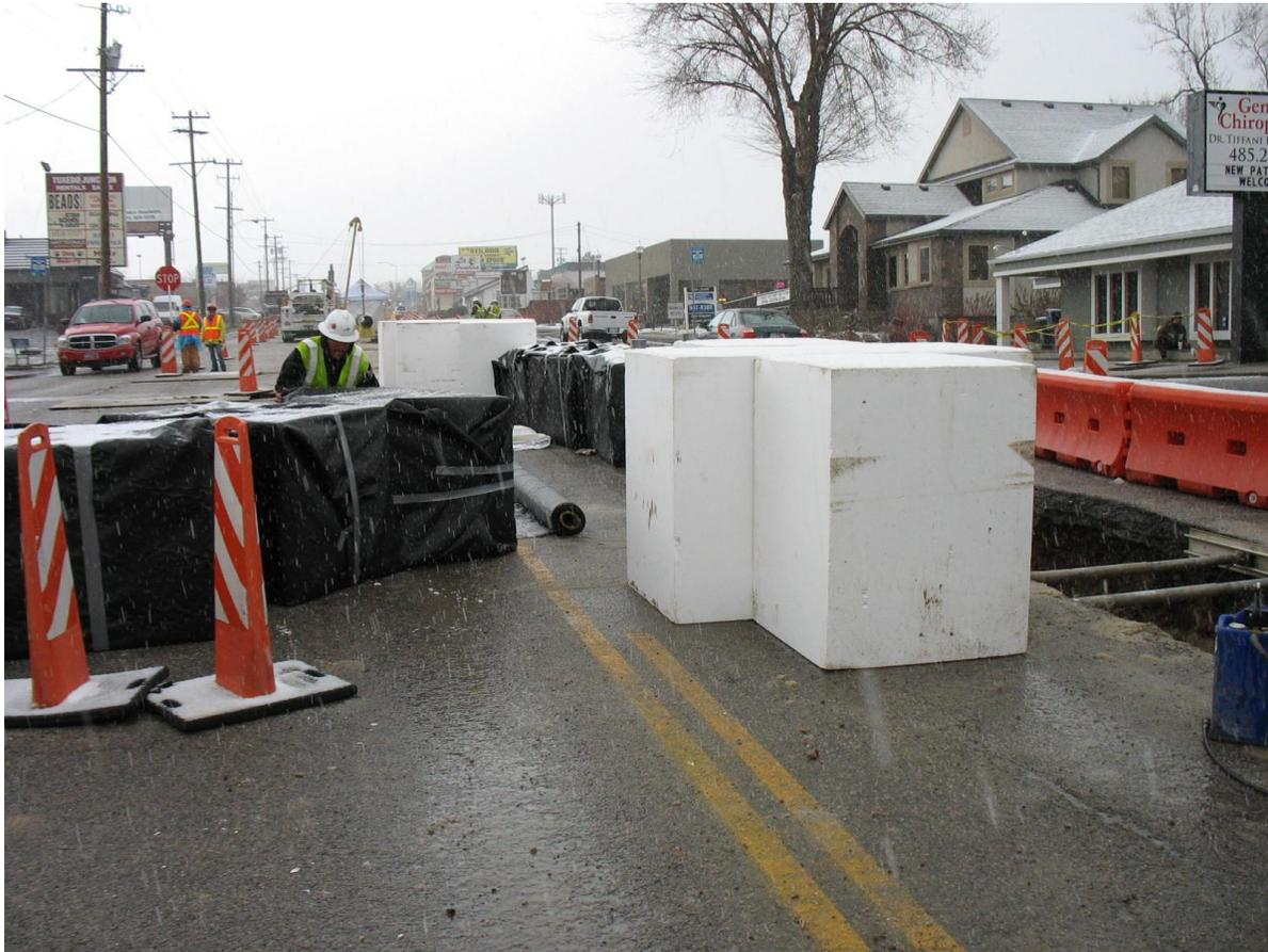
**Figure 10. Placement of geofoam block as a lightweight cover atop a 0.6-m diameter steel pipeline crossing the Wasatch fault zone in Salt Lake City, Utah.**
