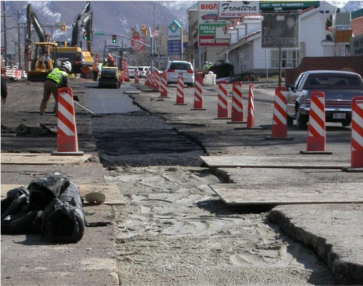
Figure 11. Placement of sand, concrete, roadbase and asphalt atop EPS cover system, Salt Lake City, Utah.
