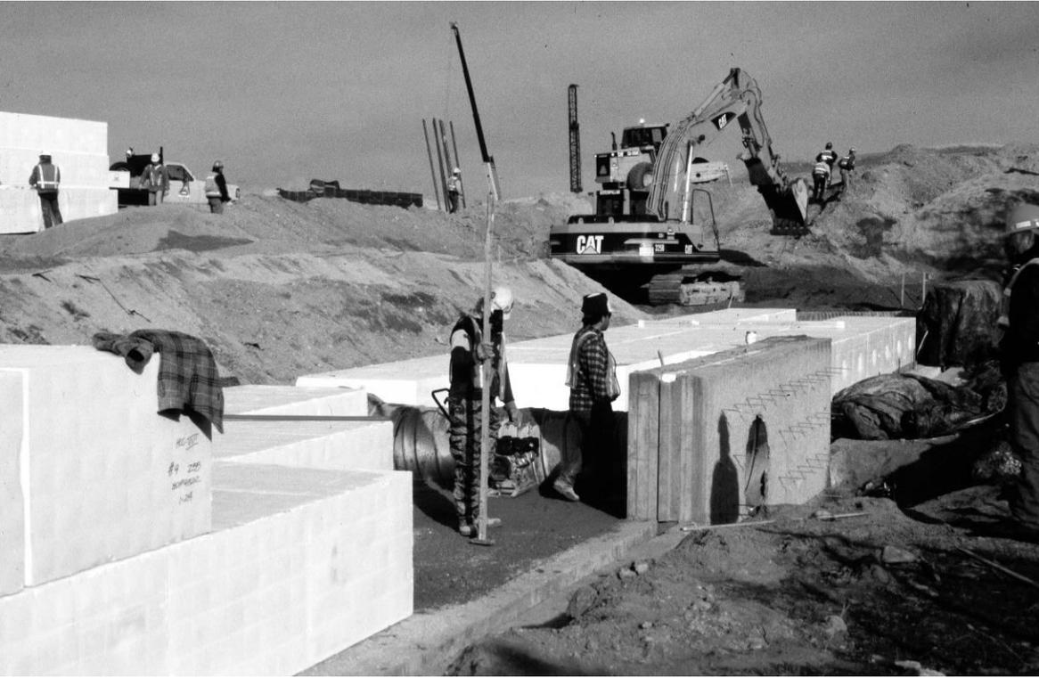
**Figure 1. Placement of expanded polystyrene (EPS) geofoam block around a steel culvert on the I-15 Reconstruction Project, Salt Lake City, Utah.**
