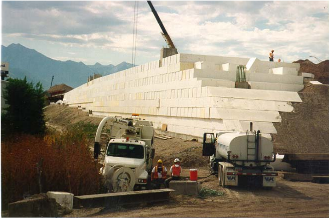
Figure 5-1 Typical Geofoam Embankment Construction on the I-15 Reconstruction Project in Salt Lake City, Utah.
