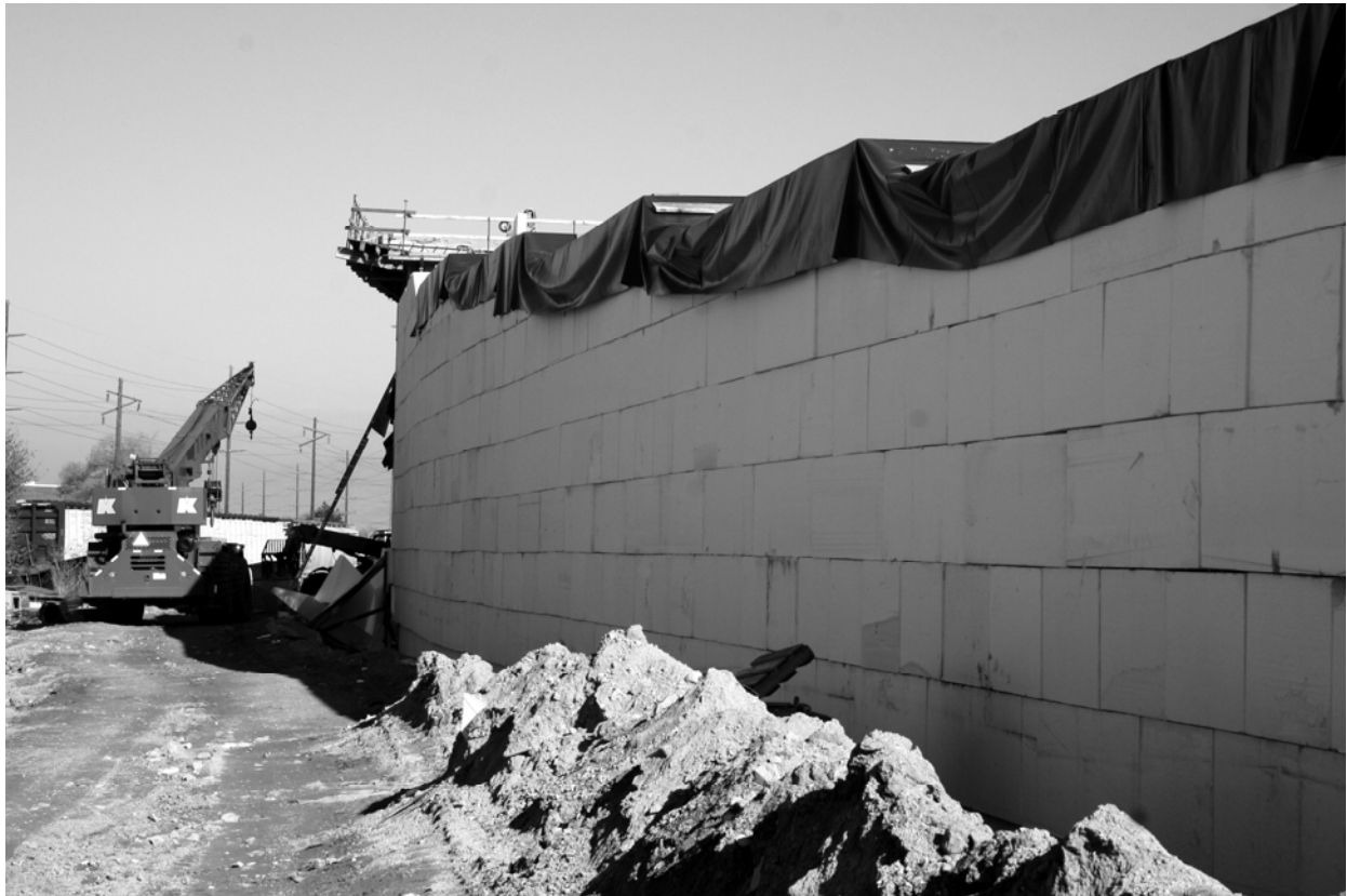
Figure 7-3 Typical Freestanding Geofoam Embankment at a Bridge Abutment.
