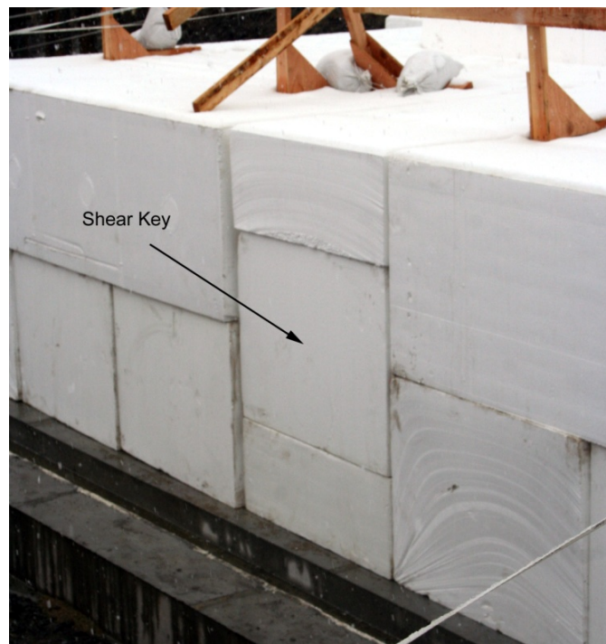
Figure 7-9 Shear Key Installed in Geofoam Embankment.
