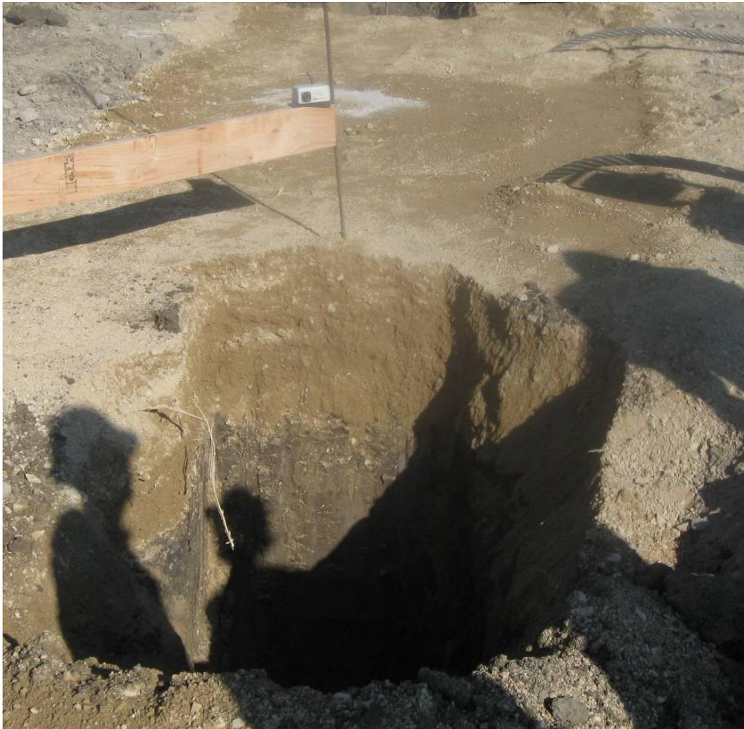
Figure 66. Soil backfill trench, with compacted fill
