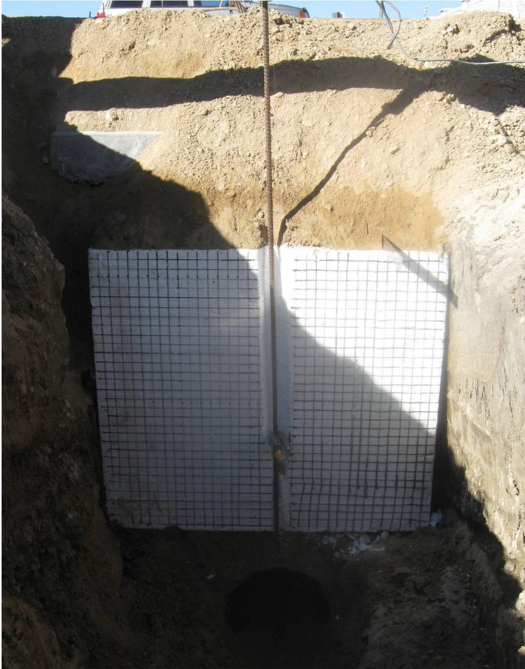
Figure 67. EPS Geofoam backfill trench
