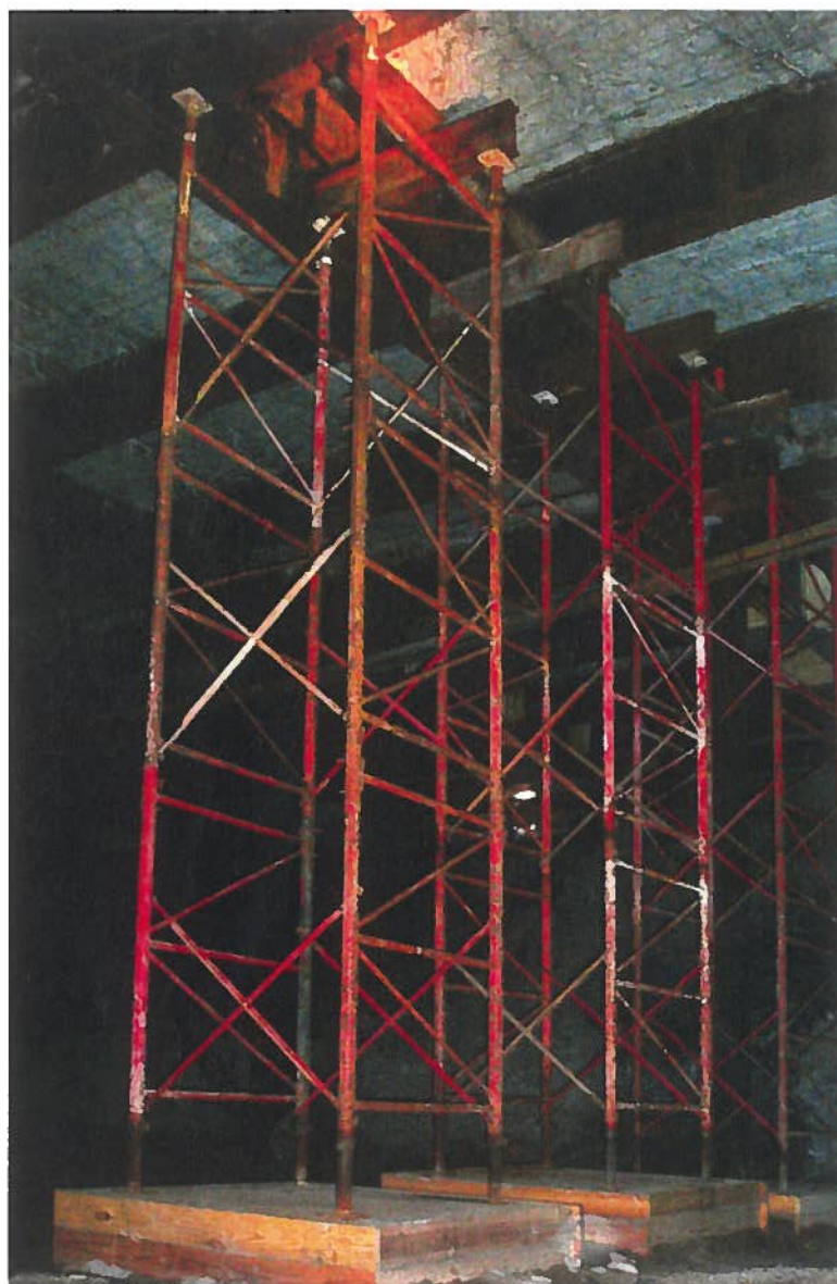
Before the reconstruction, the city used temporary shoring to support the failed ends of beams as a cost-effective way to keep the bridge open as long as possible.
