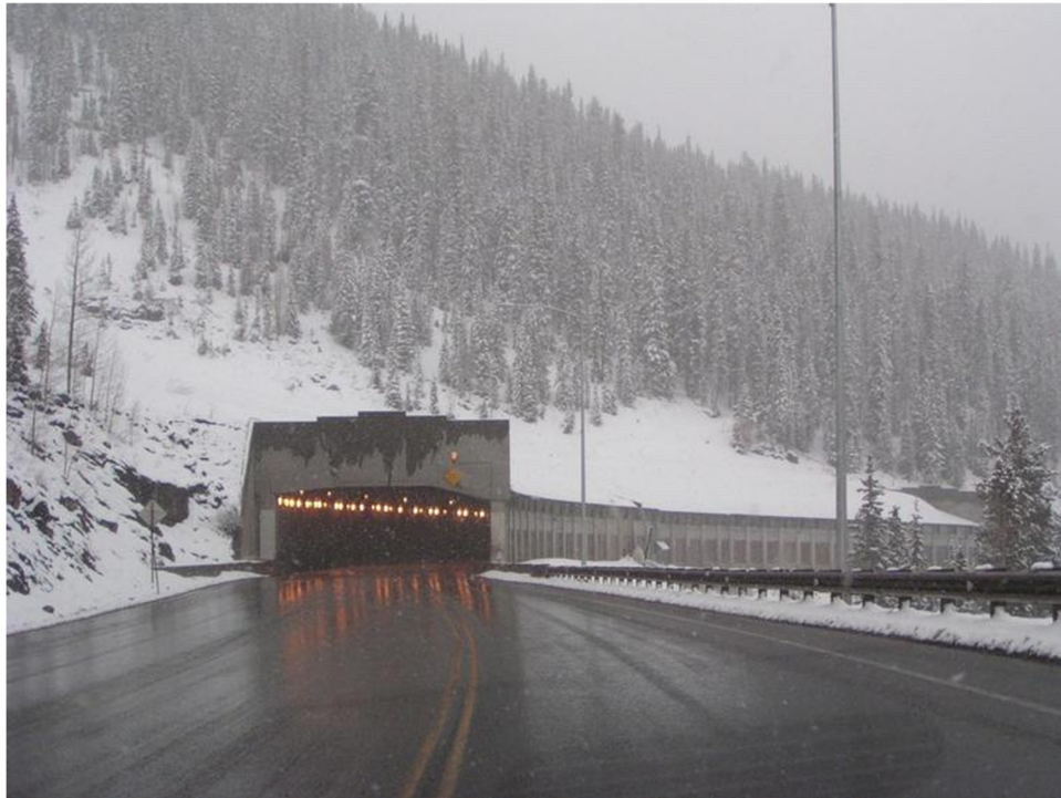
Figure 15 – Typical concrete box culvert (snow shed) in an avalanche-prone area
