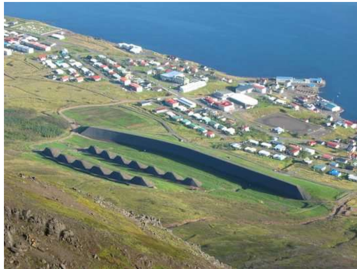
Figure 1. Two braking mounds and a catching dam at the bottom of the slope to protect Neskaupsstaður, Iceland.
