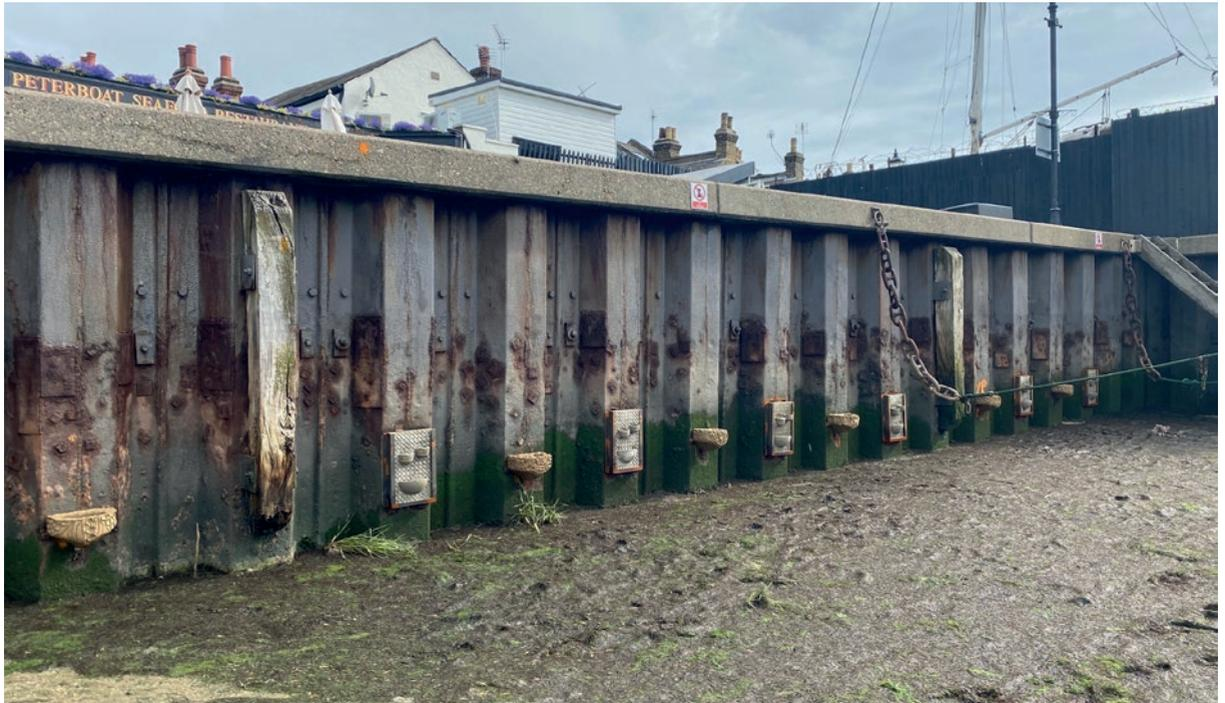
**Vertipools and steel piling habitats.** Small pools of low-carbon materials such as quarry waste provide an ideal substrate for marine life.
