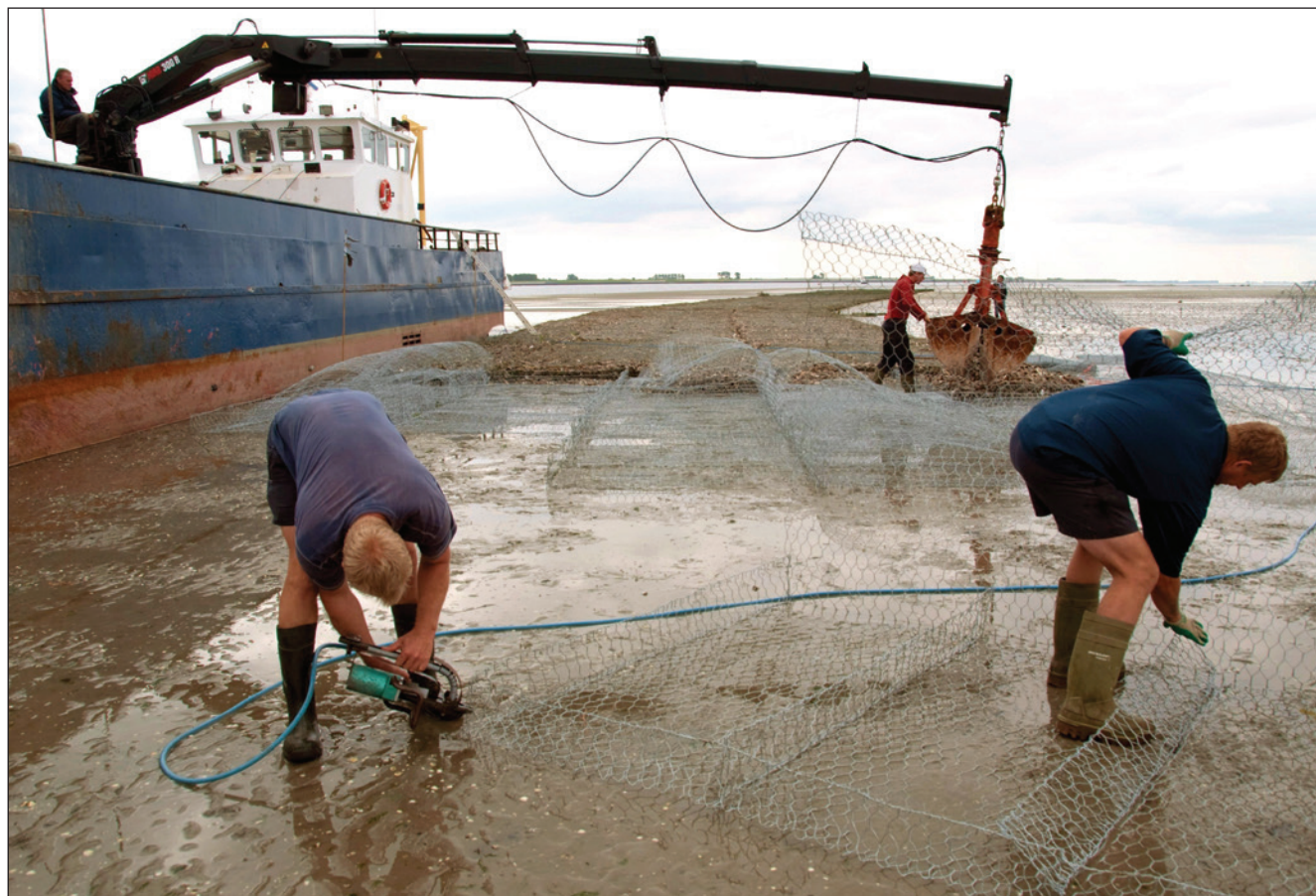
Figure 3. Oosterschelde oyster reef under construction – old oyster shells in steel wire gabions are placed as a substrate (courtesy Tom Ysebaert)
