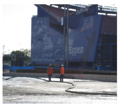
AQUAERiX permeable low-density cellular concrete was installed as a sub-base under the playing field at Citi Field, home of the NY Mets, to facilitate drainage, replacing the 4 feet of lightweight aggregate listed in the original spec saving the owner time and cost.
