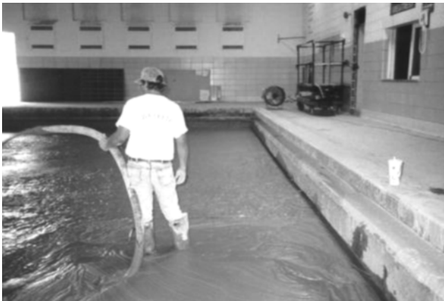
Fig. 7.5—Filling abandoned swimming pool with low-density concrete.
