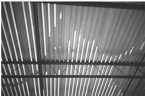
Fig. 6.1—Casting cellular concrete over vented steel deck.
