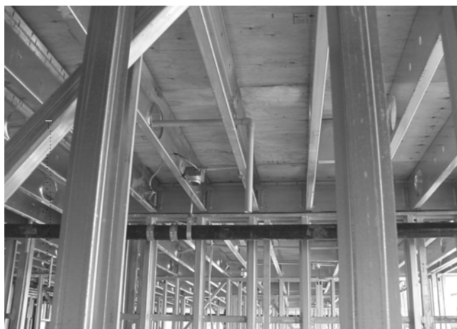
Fig. 6.4—Wood frame roof deck substrate from below.
