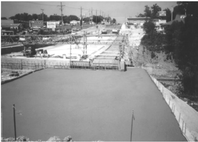
Fig. 7.3—Geotechnical roadway base at bridge approach.
