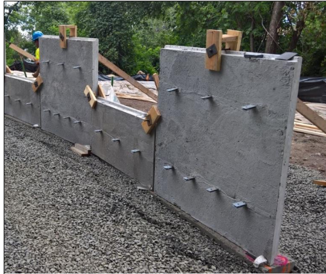
Figure 2. Offset-Alternate Panel Arrangement with Panel-to-Panel Bracing
