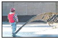
Cellular Concrete has been pumped over 700 feet vertically and over 15,000 feet horizontally
