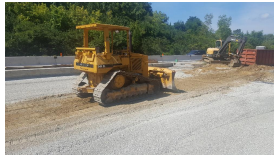
Sinkhole remediation in the median
