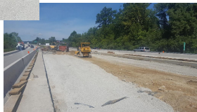
Sinkhole remediation in the median
