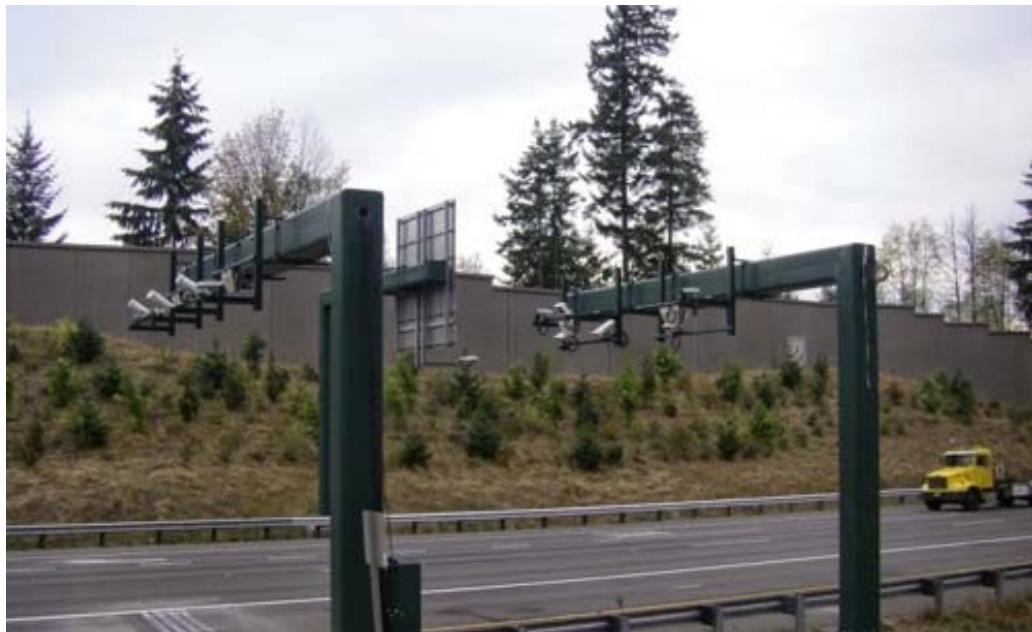
Figure 13 – Gantry and cameras for user fee assessment
