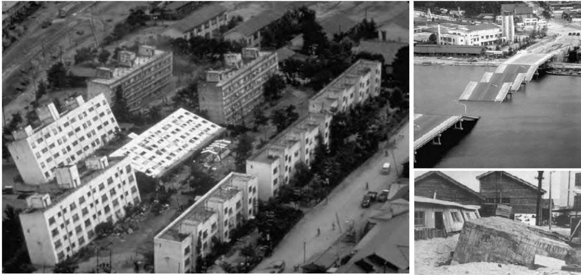
Figure 1.1. Examples of soil liquefaction consequences on human-made structures (Idriss & Boulanger 2008).
