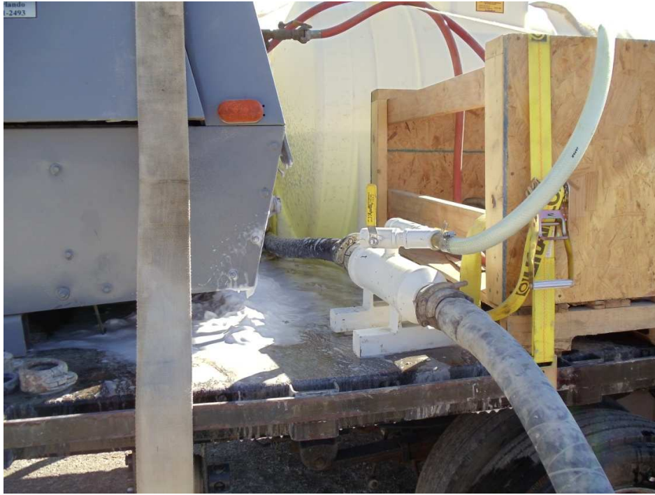
Figure 5 – Injection of Foam into the Cement-Slag Slurry to Form CLPC
