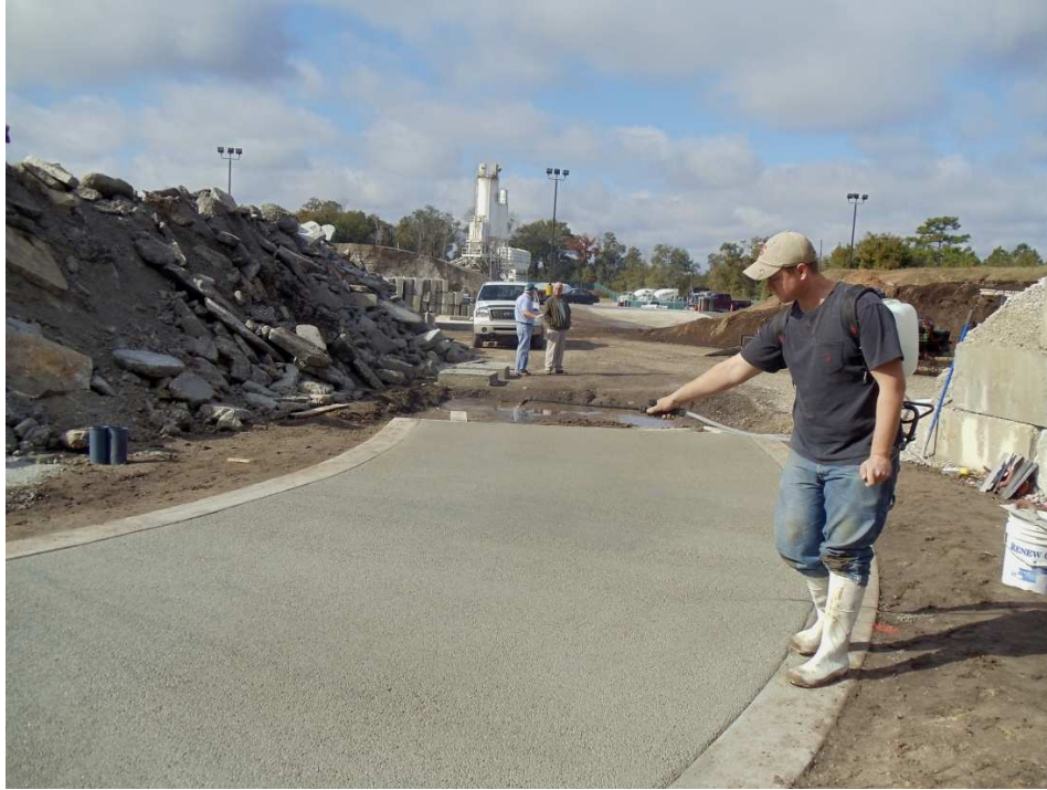
Figure 9 – Spraying Surface with Lithium Cure
