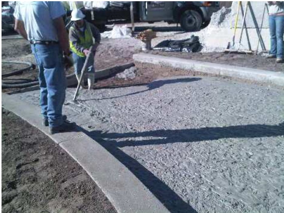
Figure 6 – Pumping CLPC Base
