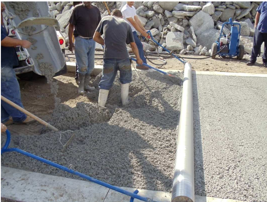
Figure 8 – Placement and Compaction of Pervious Pavement
