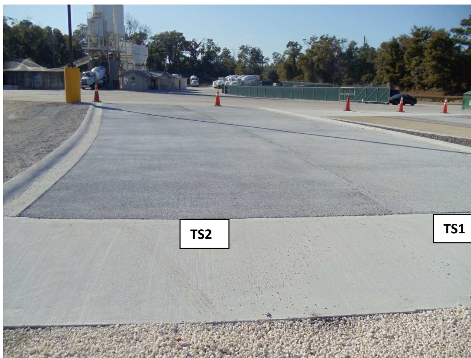
Figure 2 – Test Sections 1 (plastic sheet cure) and 2 (Lithium Cure) on aggregate base.
