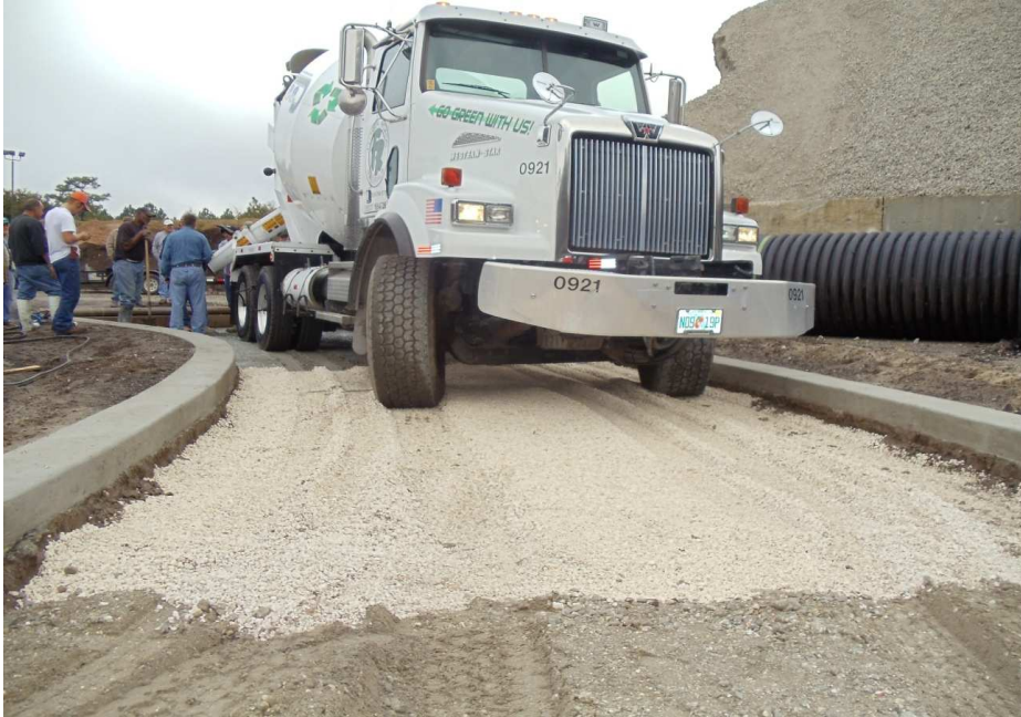
Figure 7 – Ruts in Base Layers Caused by Heavy Truck Mixer
