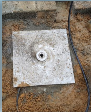
Settlement Gauge Installation
