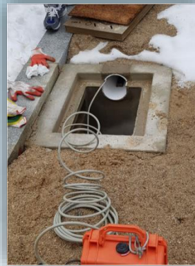
Flow Meter Installation
