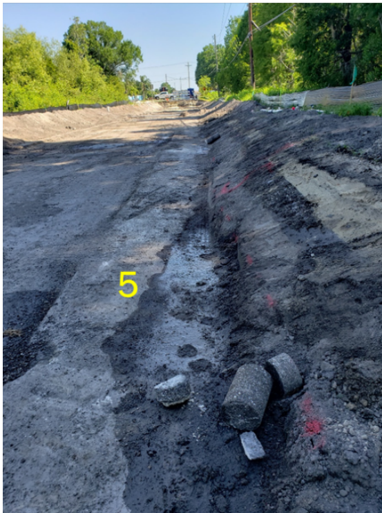
Figure 4 Existing and Prior Layers of Asphalt Ex. 2, West Lake Eloise Drive
