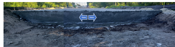
Figure 7 Water Filtration through PLDCC, West Lake Eloise Drive
