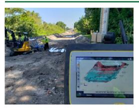
The remediation of West Lake Eloise Drive began with dewatering the jobsite, which involved the placement of well pipes along the 470-foot-long portion of roadway. The well pipes were driven twelve feet underground and spaced six feet apart along both sides of the roadway. While dewatering was in progress, the roadway was excavated and all existing material was removed, including all layers
