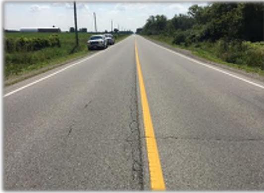
Longitudinal Cracking (centreline)
