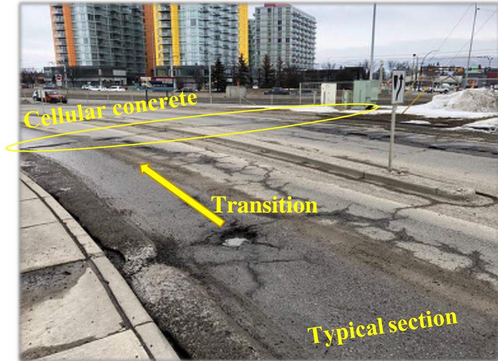
Figure 3-13: Pavement Distresses on the non-LCC section - 1(CEMATRIX, 2018)
