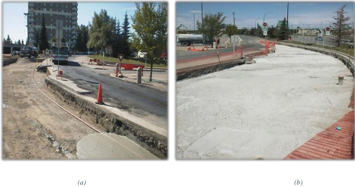
Figure 3-12: Bus Lane. (a) Reconstruction Process. Placing the LCC (CEMATRIX) (b) After Installing the LCC Layer (CEMATRIX)
