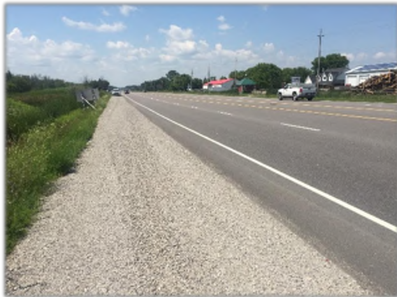
Figure 3-22: Condition of Highway 9, Three Years after Construction
