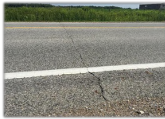
Transverse Cracking
