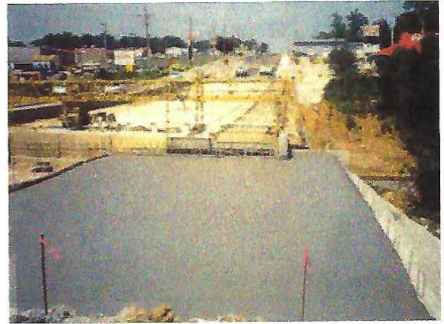
Fig. 9.2.2—Geotechnical roadway base at bridge approach.
