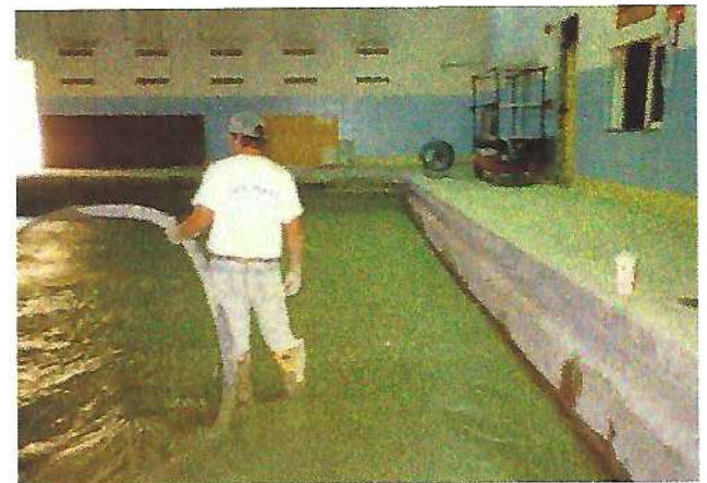
Fig. 9.2.4—Filling an abandoned swimming pool with LD-CLSM.
