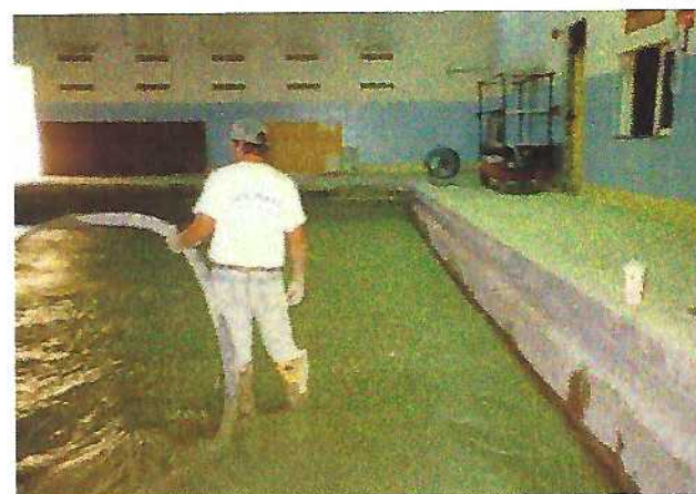
Fig. 9.2.4—Filling an abandoned swimming pool with LD-CLSM.
