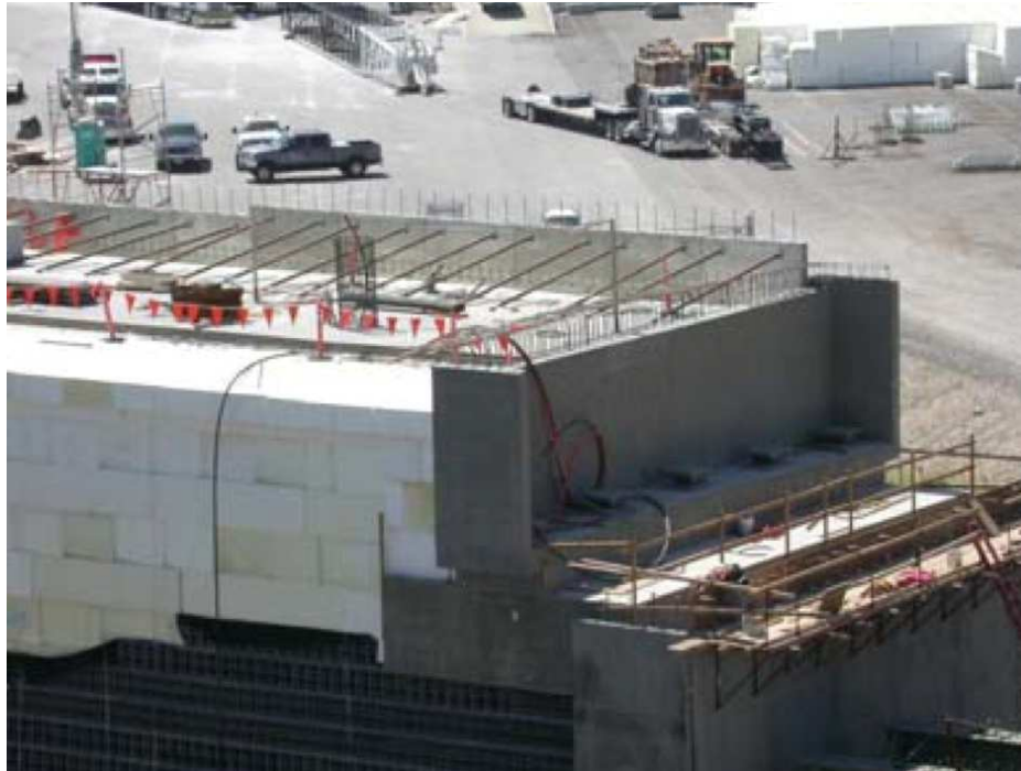
Figure 1.7 Geofoam at UTA TRAX Light Rail
