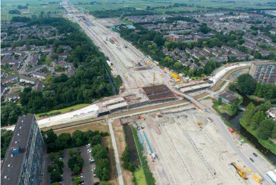
Figure 1.9 EPS Embankment in Netherlands
