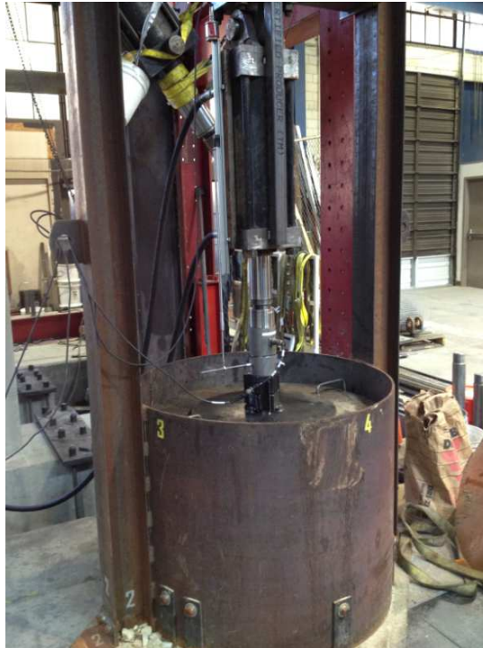
Figure 3.3 Completed Test Set-up
