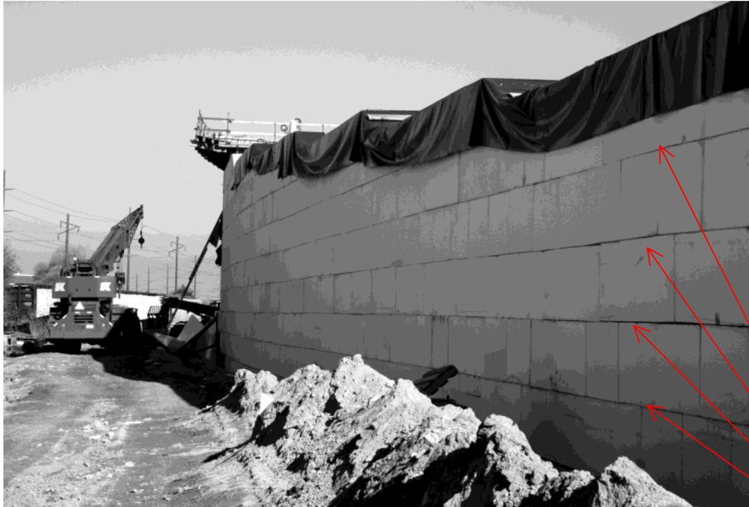
Typical freestanding geoforembankment at bridge approach. Note that continuous horizontal planes are created by the block placement pattern. **Question: Could sliding occur along these interface planes during a major earthquake?**
