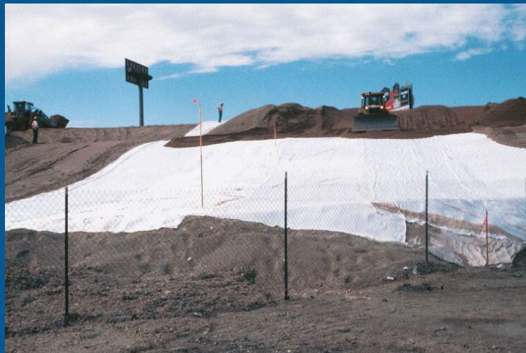
Geotextile Reinforced Slopes
