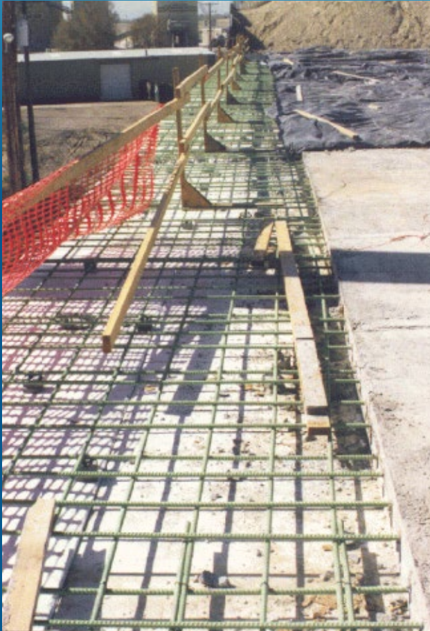
Reinforced Concrete Load Distribution Slab
