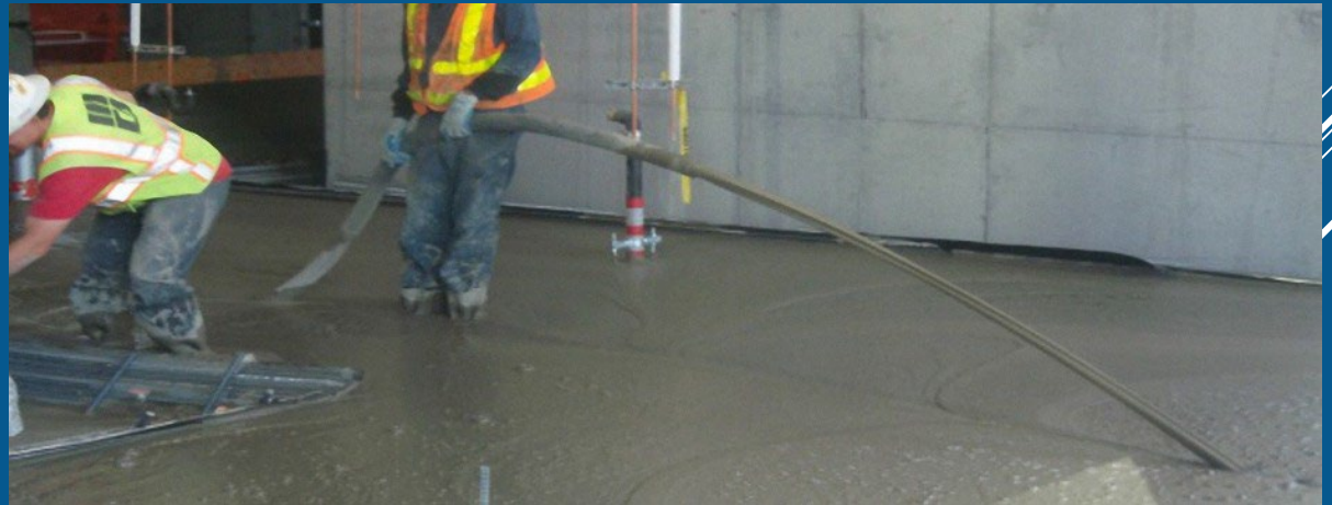
Cellular Concrete Placement photo courtesy of Aerix Industries
