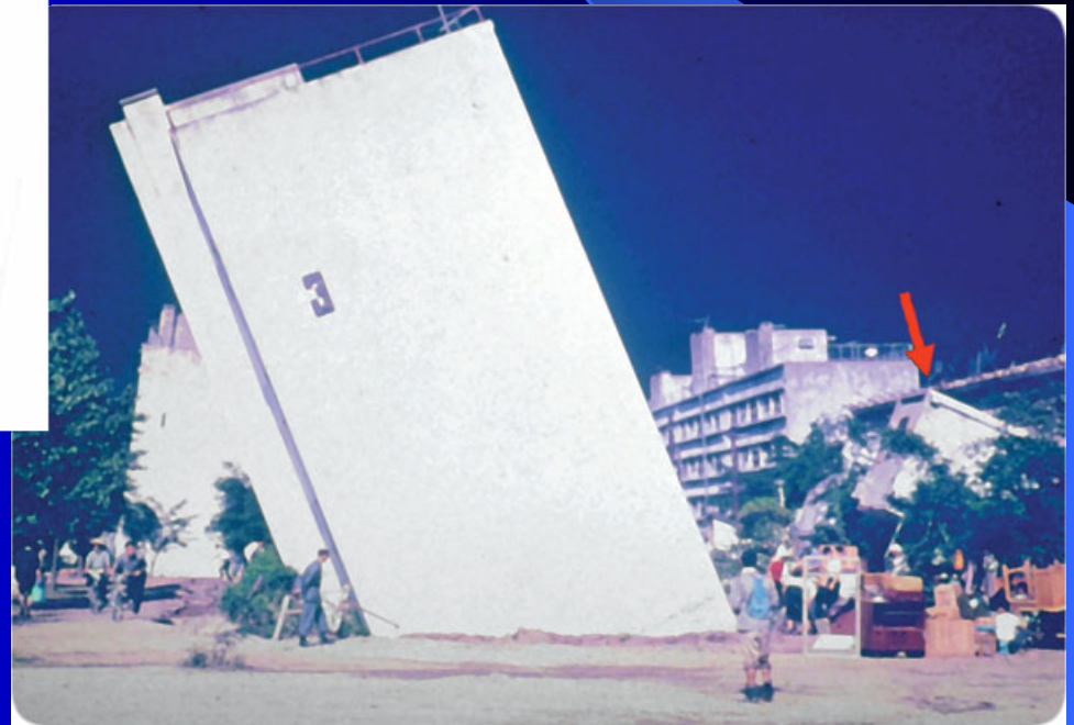
1964 Niigata, Japan Earthquake
