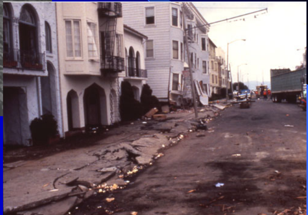
Marina District, San Francisco, 1989 Loma Prieta Earthquake
