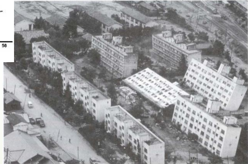
Dynamic: Foundation failure by liquefaction after the 1964 Niigata Earthquake. (USGS)
