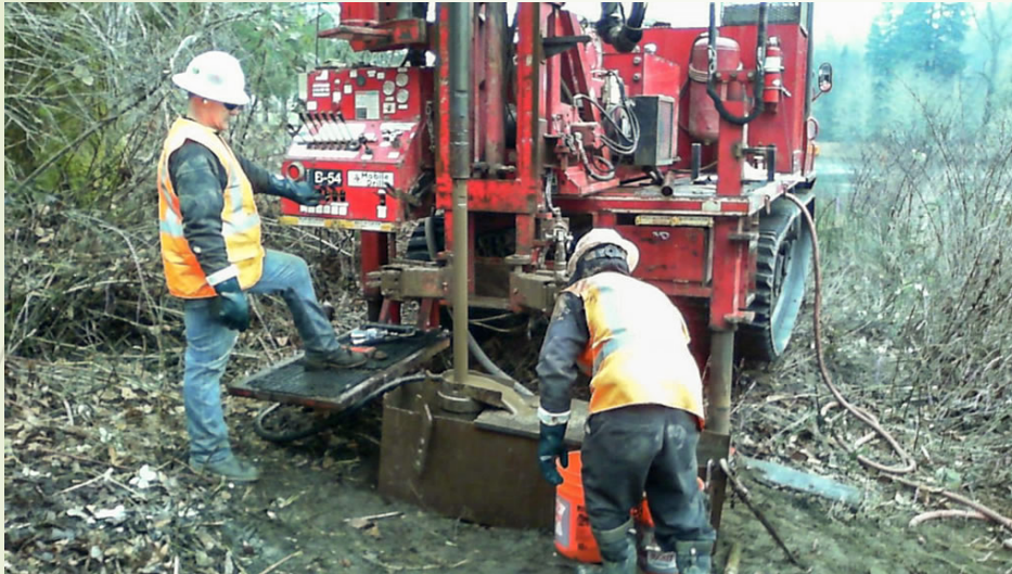
Mud Rotary Drilling
