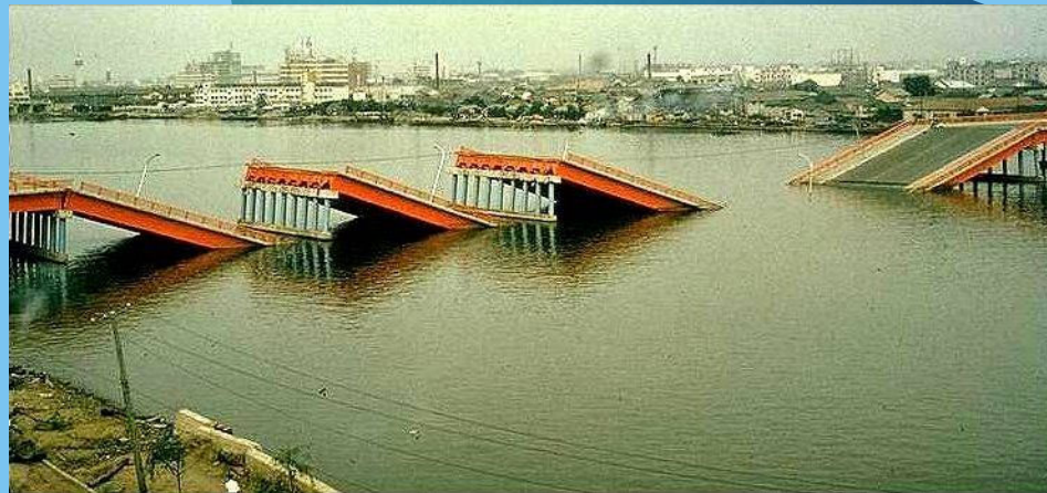
1964 Niigata, Japan Earthquake
