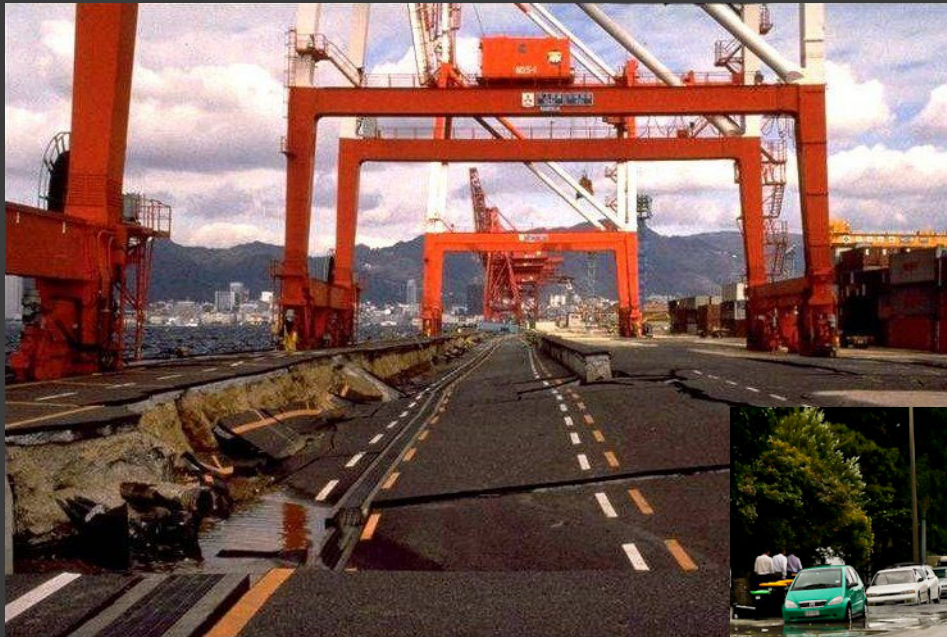
Port of Kobe, 1995 Kobe, Japan Earthquake
