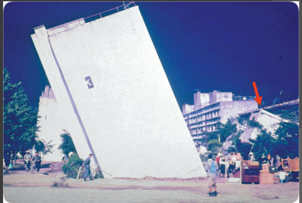
1964 Niigata, Japan Earthquake
