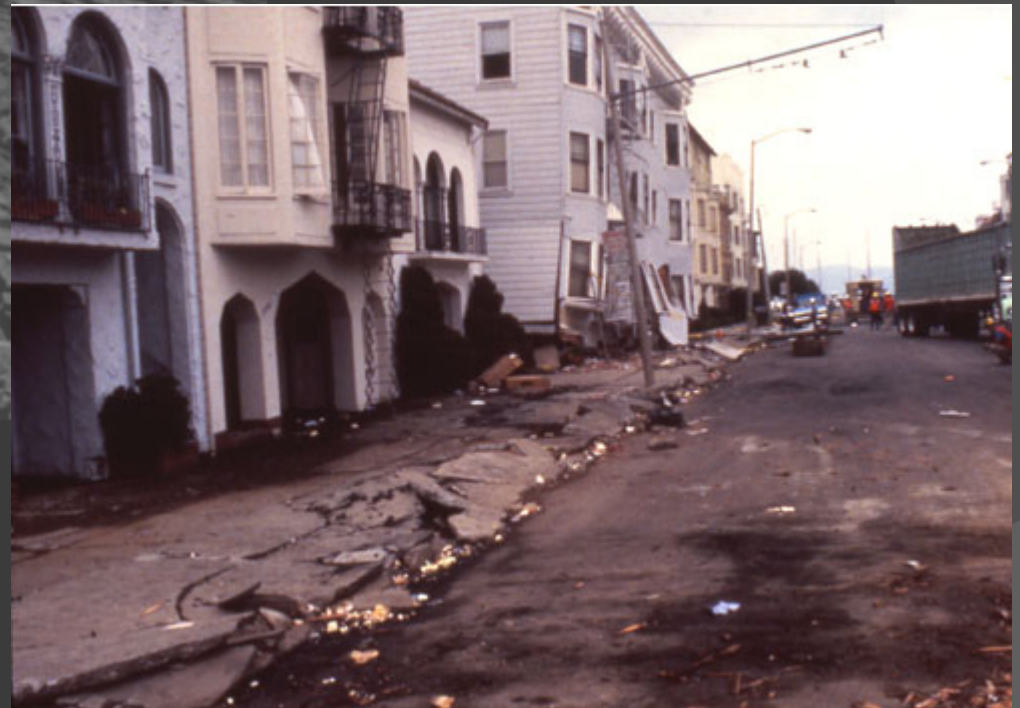
Marina District, San Francisco, 1989 Loma Prieta Earthquake
